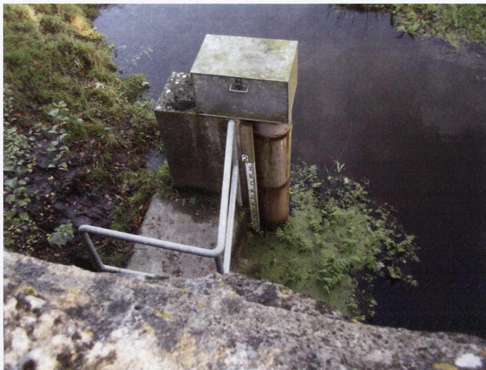
Figure 3.5a. View of the automatic data logger station for water level (Ballinarink Bridge, EPA station code 26058) and water quality sampling point located on the Ross river in the catchment draining to Lough Sheelin. Water quality samples were taken by IFI staff and automatic water level readings were monitored remotely by the EPA
