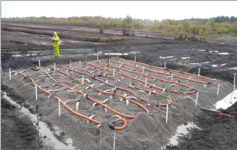
Vacuum lines, PVDs, instrumentation in place; awaiting sealing membrane cover.
