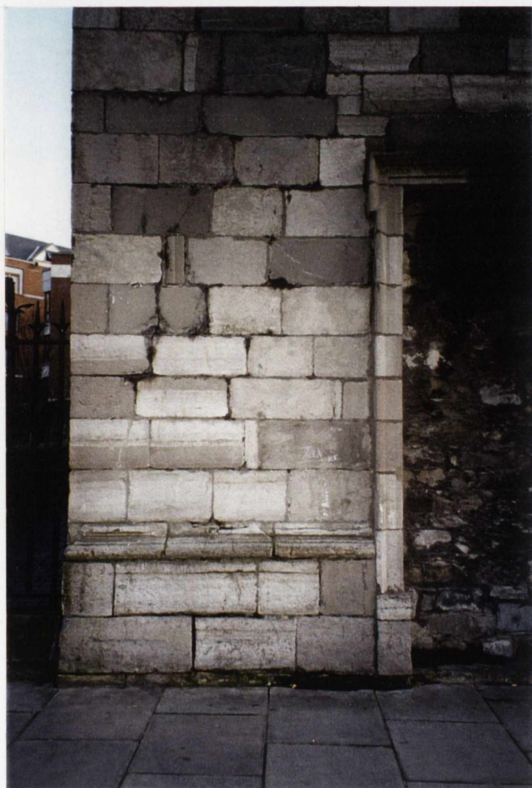
fig. 7 St. Nicholas Within, Dublin 1707: Front facade of dressed calp ashlar and compound walls of calp rubble.
