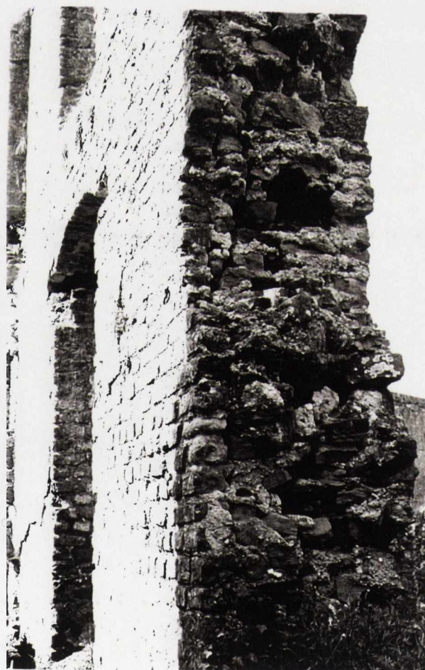
Surviving fragment of Roman compound wall in the Roman Forum (above), and a c1740's compound wall with brick internal linings at Castlestrange, Co Roscommon (below). fig
