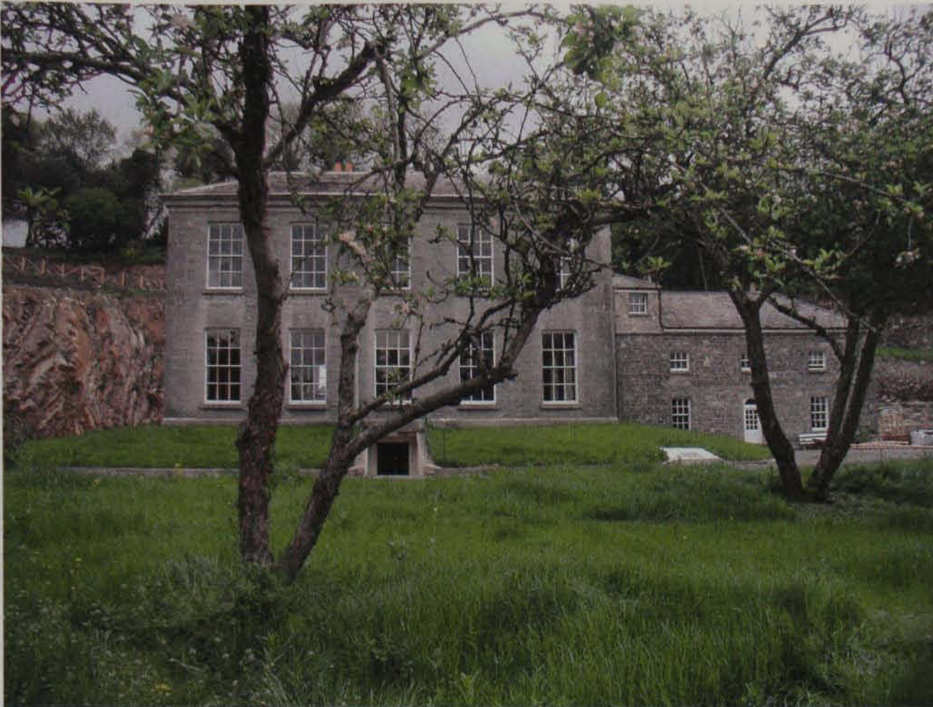
Fig.3.17: David Jebb's house called 'Janeville' facing out onto the River Boyne. The earlier building, built c. 1765, is to the right, and the five bay extension, built c.1799, is to the left.
