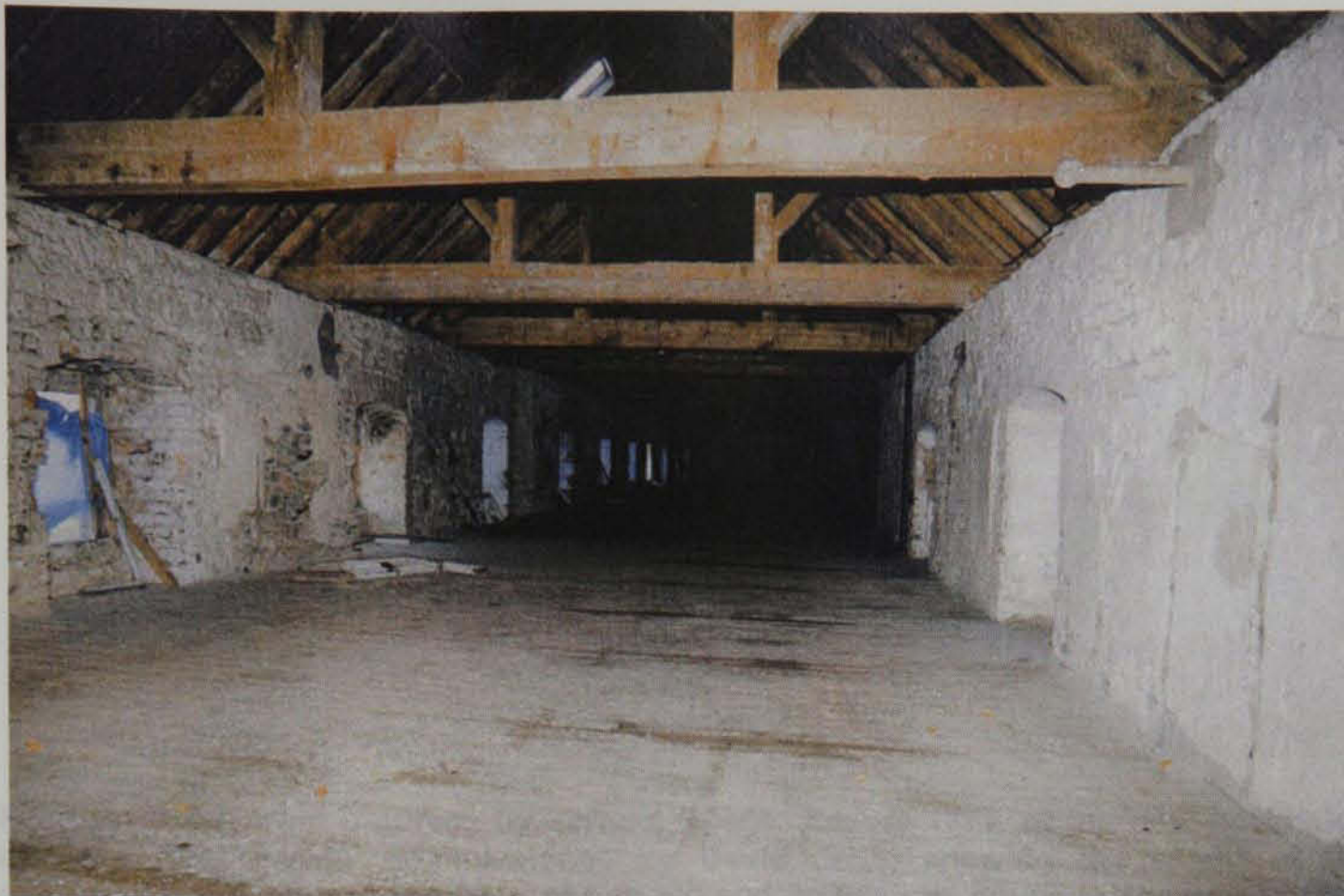
Fig.3.12: Fifth floor of the narrow block of Slane Mill, with attic level exposed. Courtesy of T.J. O'Meara, NIAH.
