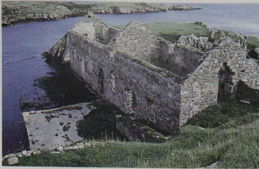
Storehouse on inlet at Corbet Hill
