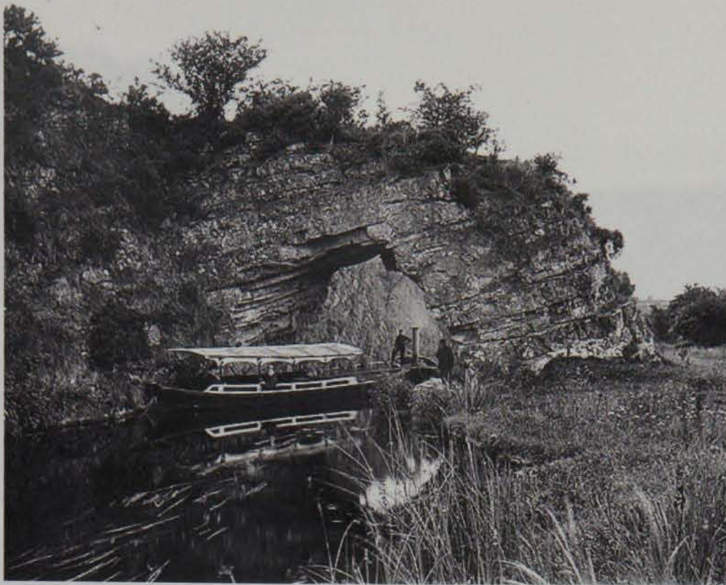
Fig. 5.14: The Rock Arch over the Boyne Navigation between Rosnaree and Slane, c. 1890. This tract of canal necessitated a large amount of rock blasting, mentioned by both Omer and Ducart in their tenders. NLI, photograph collection, LIMP 4206.
