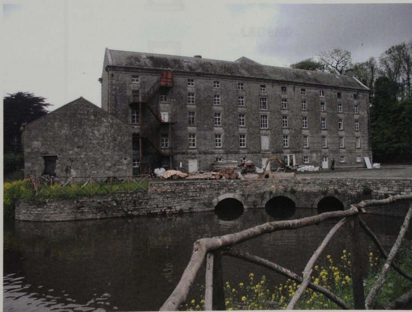
Fig.3.15: Rear elevation of Slane Mill showing the three tail-race channels exiting into the River Boyne.
