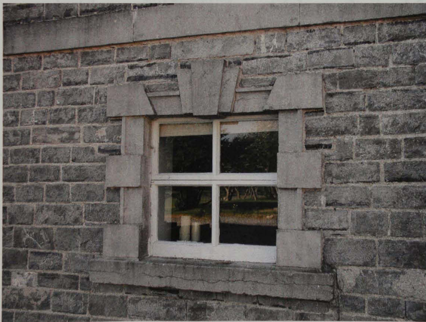
Fig.3.10: Ground floor window of Slane Mill with Gibbsian surround illustrating the contrasting stone types between the pale grey dressings and the blue-grey coursed stonework.
