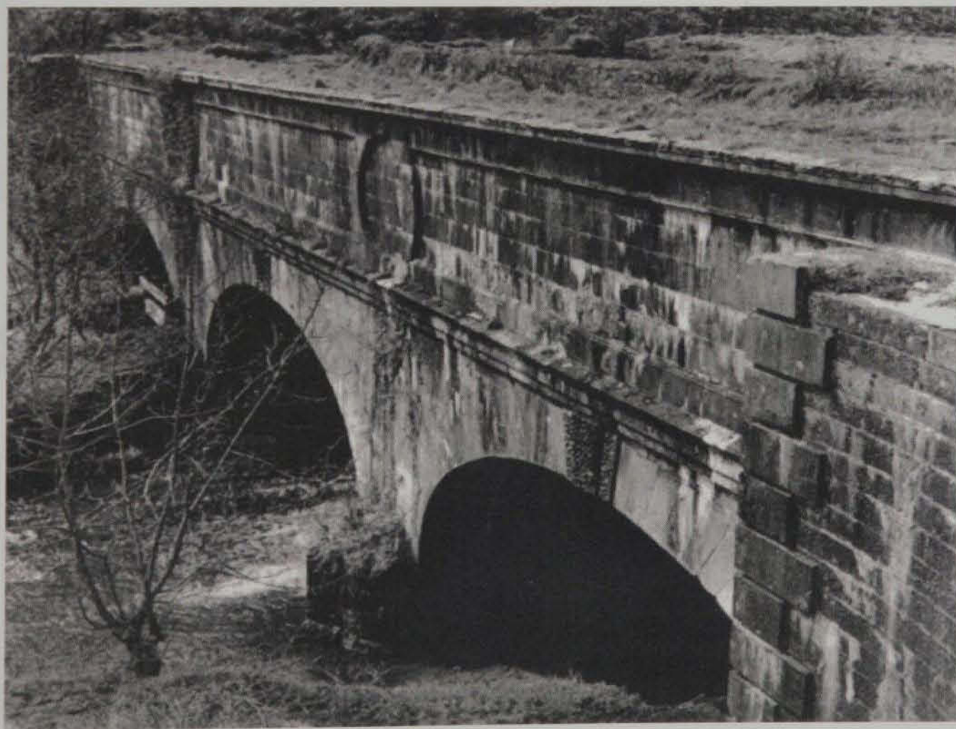
Fig. 5.17: Ducart's aqueduct at New Mills, county Tyrone. IAA, photograph collection.
