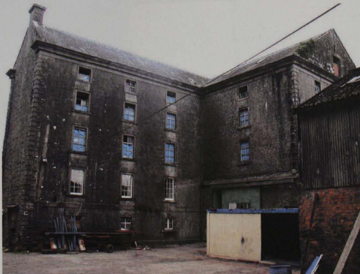
Fig.3.7: View of the mill from the north-west, taken prior to the cleaning of the stonework. Courtesy of T.J. O'Meara, NIAH.
