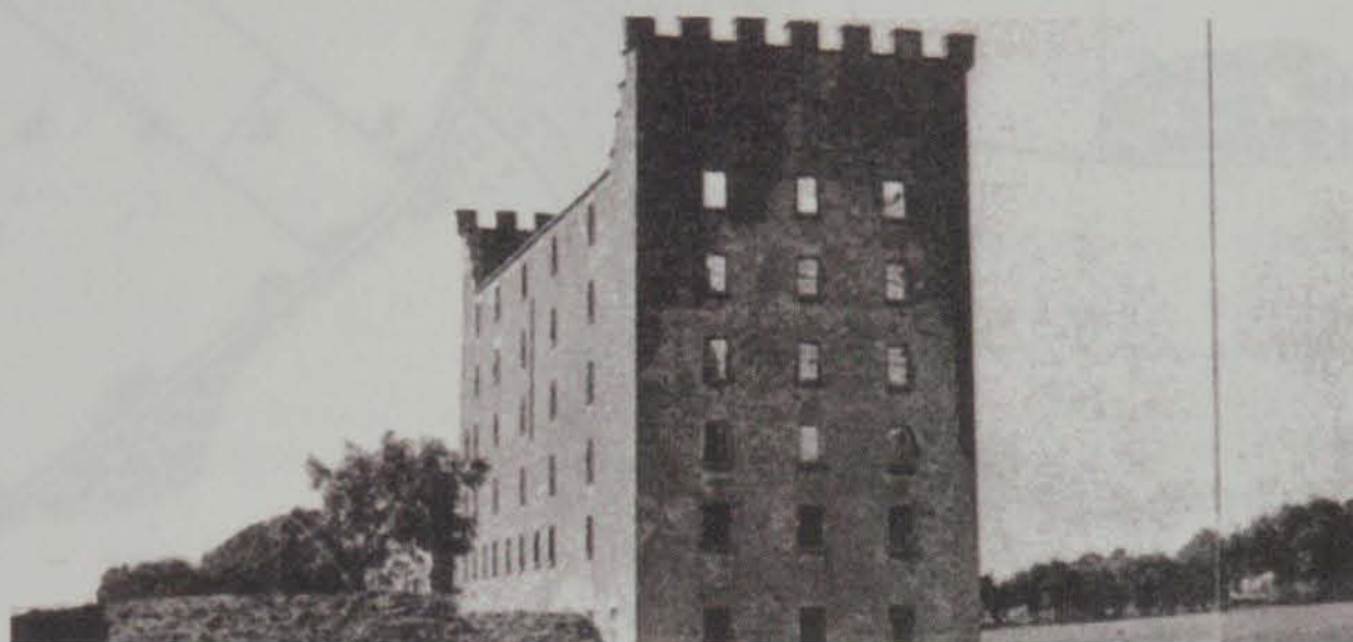
Fig.3.21: Castellated multi-storey flourmills at Milford, county Carlow (above) and New Haggard, county Meath (below). (Niall McCullough & Valerie Mulvin, A lost tradition, the nature of architecture in Ireland , Dublin, 1987).
