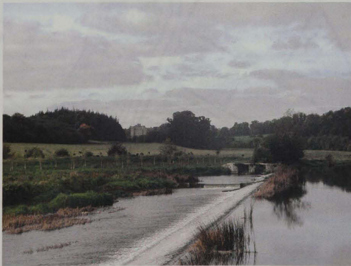
Fig.3.22: View from the mill complex across the weir towards Slane Castle demesne.
