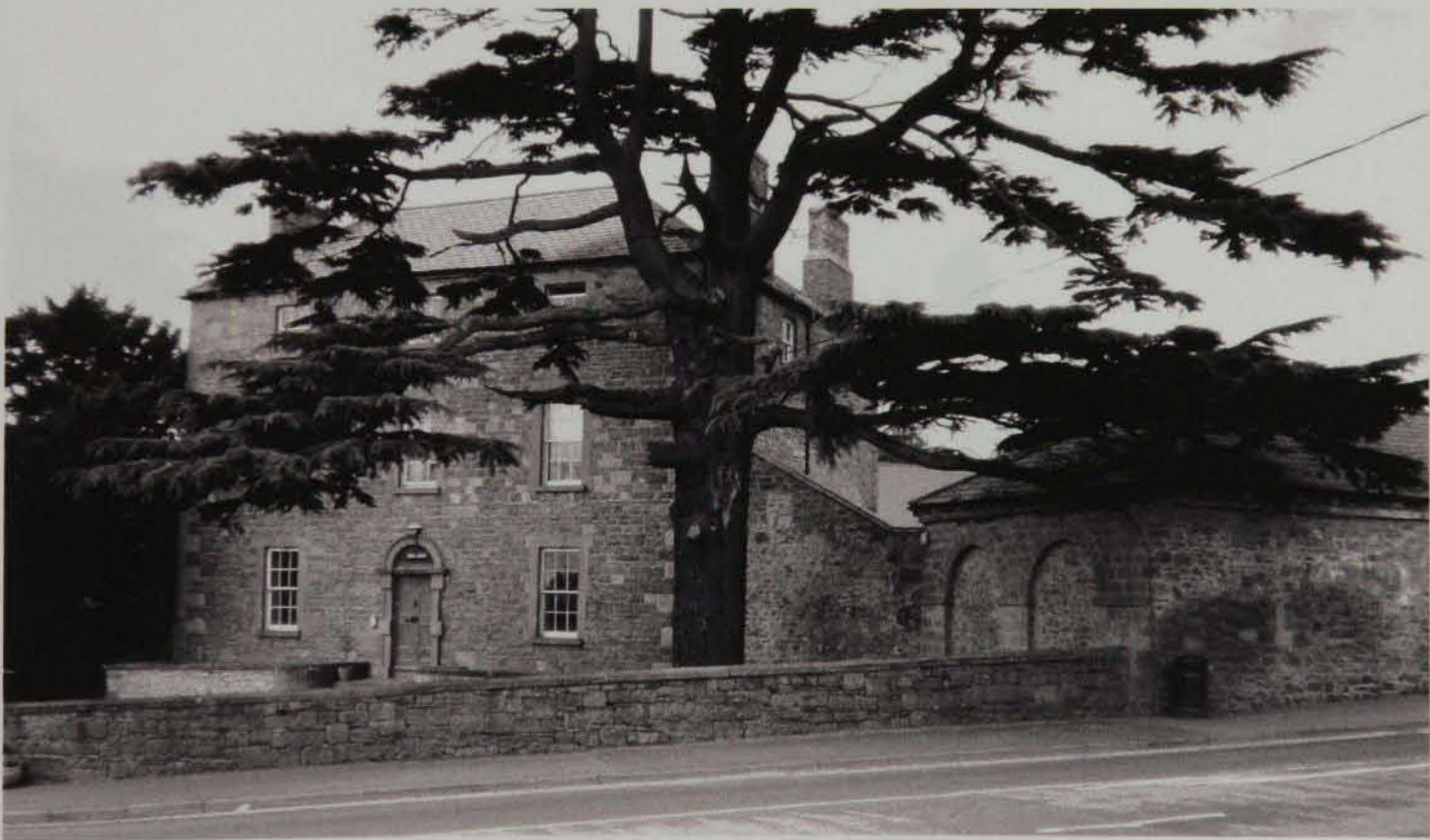
Fig.4.7: Current view of the north-western house and adjoining single-storey pavilion on Chapel Street, at Slane. The render to the blind arches has been removed revealing rubble-stone courses below the limestone surrounds.
