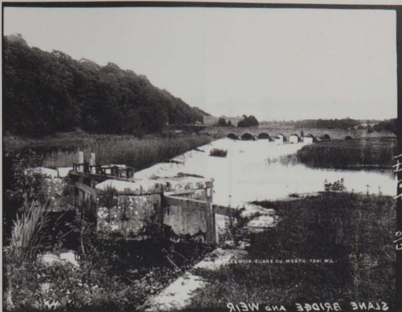
Fig.5.16: Late nineteenth-century view of the stone piers holding the floodgates as built by David Jebb. The chamfered stone detail to the piers and walls lining the riverbank mirrors that of Jebb's millpond at Slane Mill. IAA, photograph collection.
