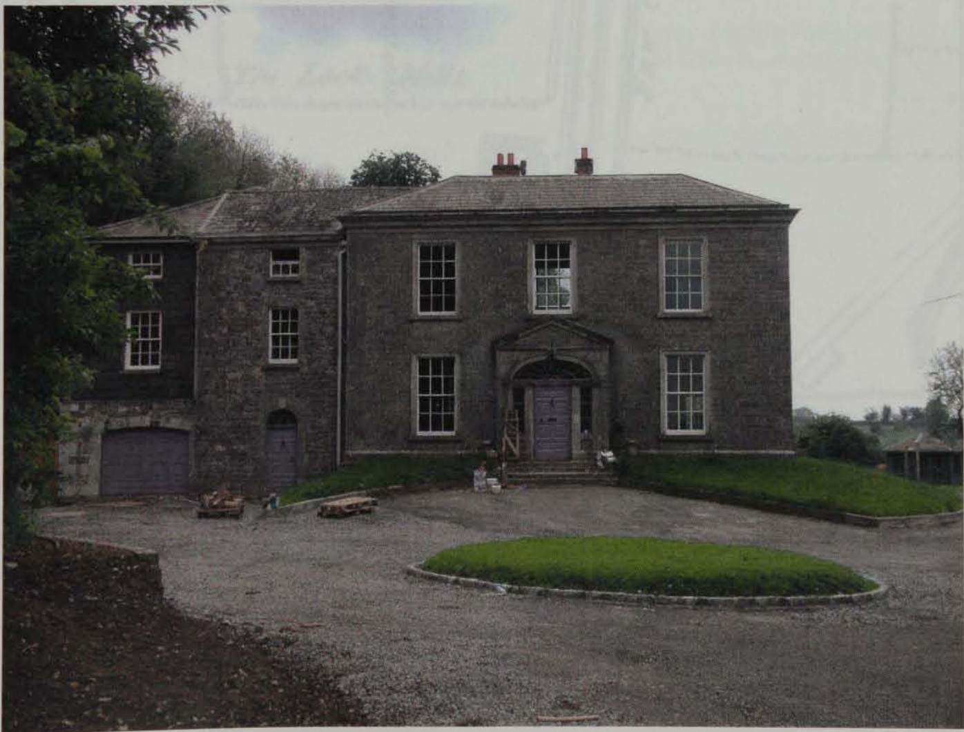
Fig.3.18: Front entrance to Janeville, built c. 1799.
