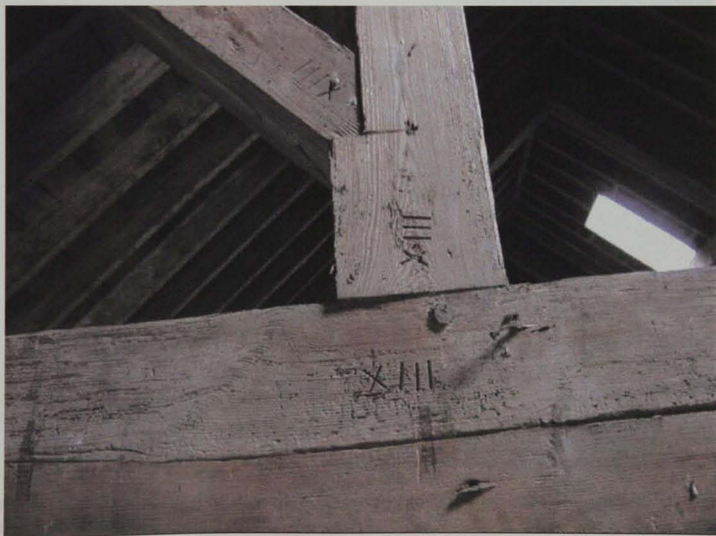
Fig.3.13: Detail of roof timbers of Slane Mill, with carpenters' marks still visible. Courtesy of T.J. O'Meara, NIAH.
