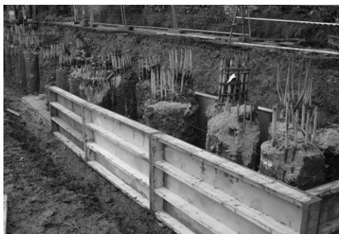
(c) Placement of formwork for construction of capping beam
