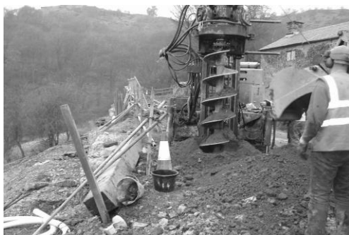
(a) Lightweight auguring rig
