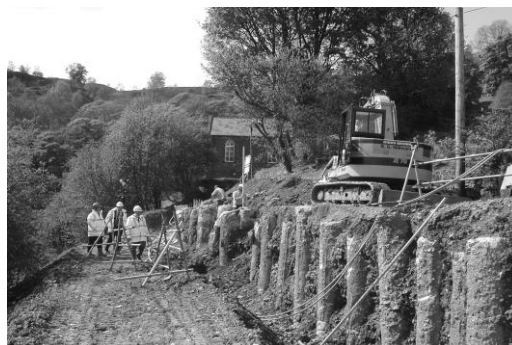
(b) Outermost row of piles
