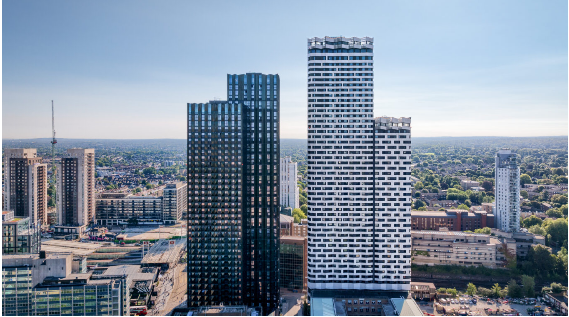
Figure 4.9: Ten Degrees and College Road , Europe’s tallest volumetric modular buildings (Source: Tide Construction [25])
