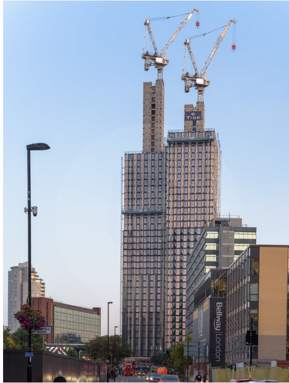
Figure 3.1: Typical volumetric modular building with RC core (Source: Tide Construction [6])
