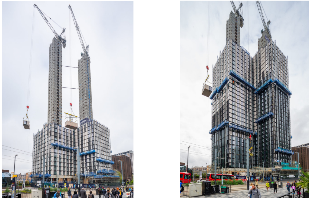
Figure 5.5: The Ten Degrees building in Croydon, London, pictured at two points in time during module installation (Source: Tide Construction [216])
