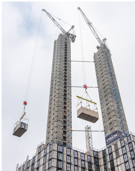
Figure 1.1: Example of modules being lifted into place in the Ten Degrees project in Croydon, London (Source: Tide Construction [6])
