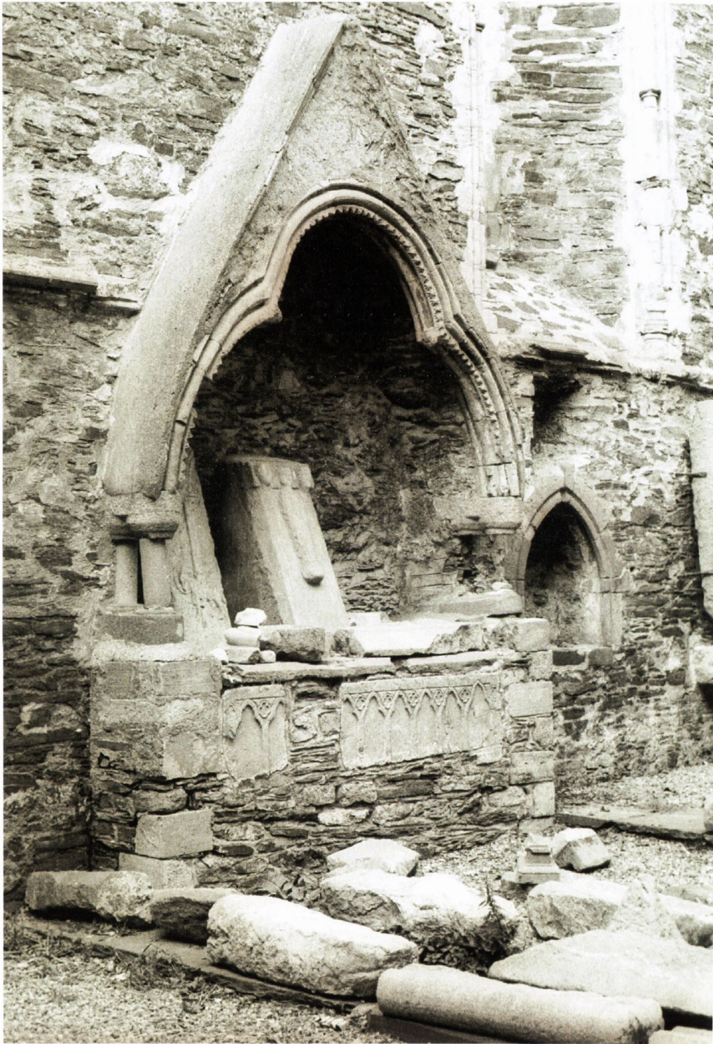
Image 2.11 Tomb niche, thirteenth century, north elevation of chancel, St Mary's parish church, New Ross, Co. Wexford [image from TARA, Stalley Collection http://hdl.handle.net/2262/39436 ]
