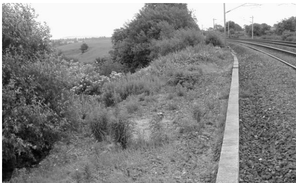
Figure 3. View southwards along Up-line slope.
