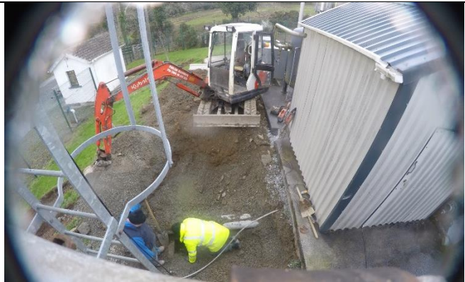
b) Excavations to expose the pipeline
