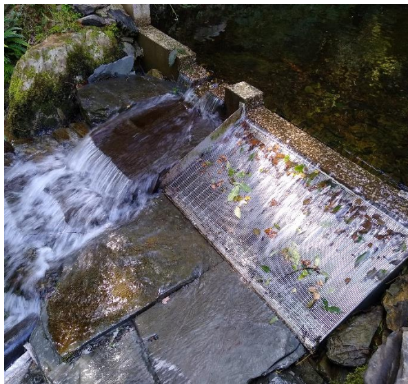
FIGURE 7-10. CONSTRUCTION OF THE WATER INTAKE STRUCTURE: A) AND B) POSITIONING OF THE PRE-CAST CONCRETE WEIR INTO THE STREAM; C) AND D) AFTER RESTORATION OF THE RIVER BED AND CONNECTION TO THE PIPELINE.
