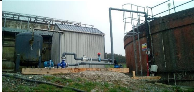
FIGURE 7-38. PROGRESS OF FIELD WORK: A) INITIAL SITUATION; B) EXCAVATIONS TO EXPOSE THE PIPELINE; C) INSTALLATION OF A RISING TEE; D) CASTING OF THE CONCRETE SLAB EXTENSION; E) TURBINE INSTALLATION; F) FINAL PIPE LAYOUT.
