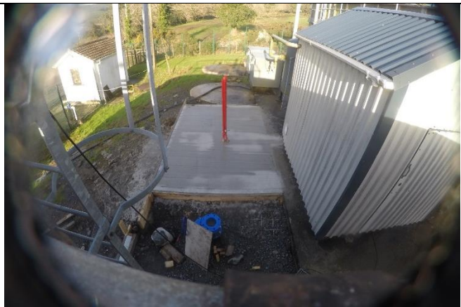
d) Casting of the concrete slab extension
