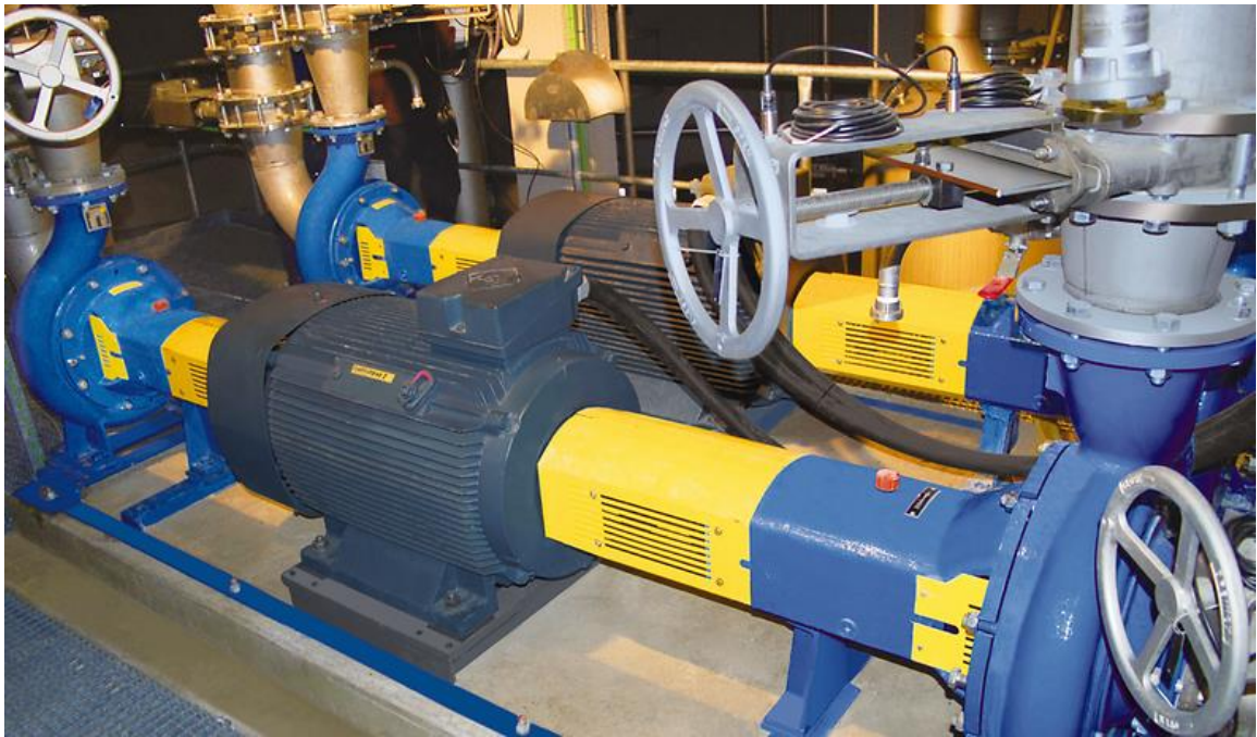
FIGURE 3-40. ENERGY RECOVERY INSTALLATION USING A PAT AT A PAPER MILL IN GERMANY (ANDRITZ, 2018).
