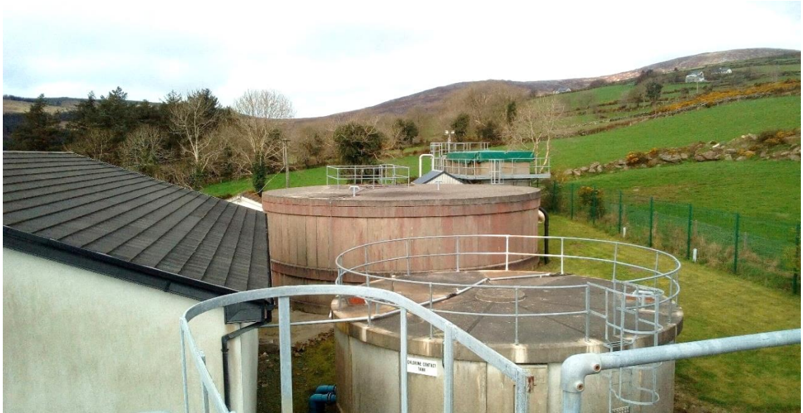
FIGURE 7-23. OVERALL VIEW OF THE BLACKSTAIRS WATER TREATMENT PLANT.
