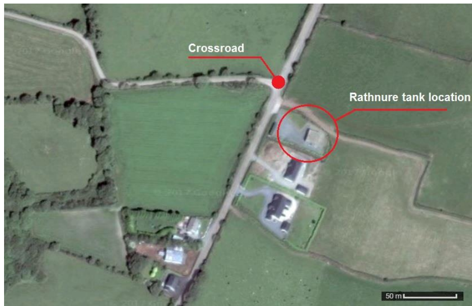
FIGURE 0-46. AERIAL VIEW OF THE RATHNURE TANK AND THE NEARBY CROSSROAD
