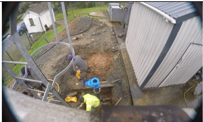
c) Installation of a rising tee
