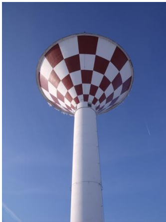
FIGURE 3-9. ELEVATED CONCRETE-MADE WATER TOWER AT SCURZOLENCO (IT).
