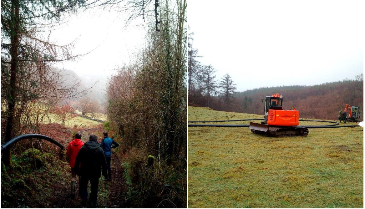
FIGURE 7-11 - LAYING OF THE 6" PIPELINE FROM THE SOURCE TO THE POWERHOUSE.
