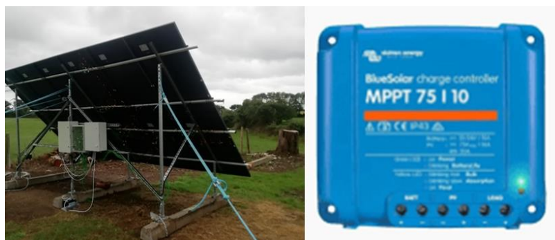
Figure 1-24: Solar test site Left: The rear of a solar panel array, Right: A maximum power point tracker
