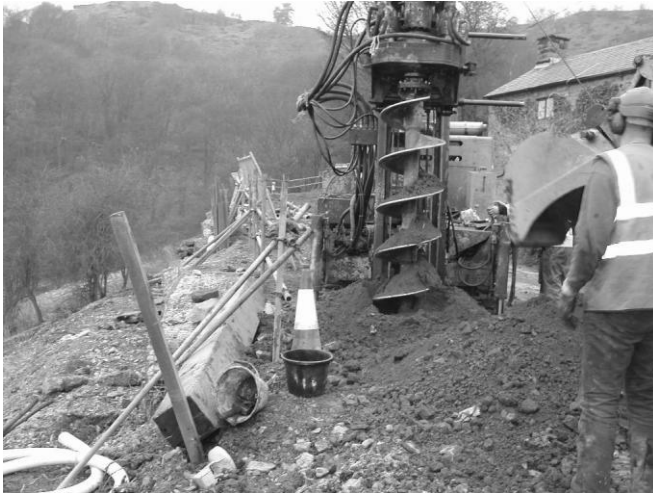
25-tonne compact Bauer rig
