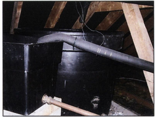
b) CWS prior to upgrading
