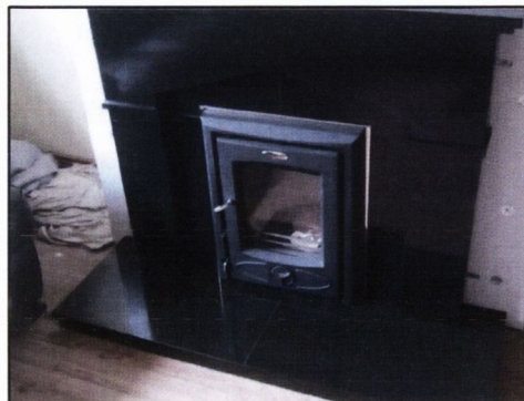
Figure 41 Stanley Cara Insert Stove and surround fit at Dwelling D
