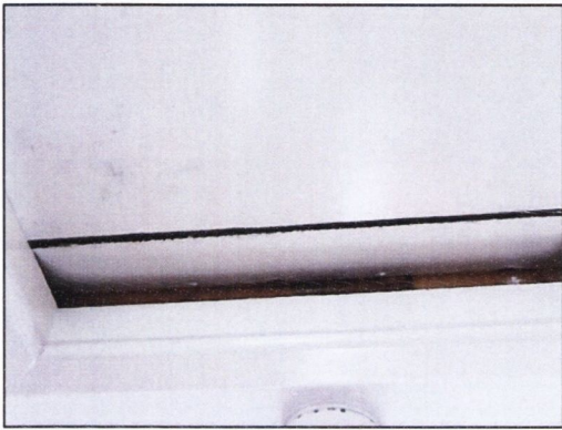
c) Attic hatch prior to upgrading
