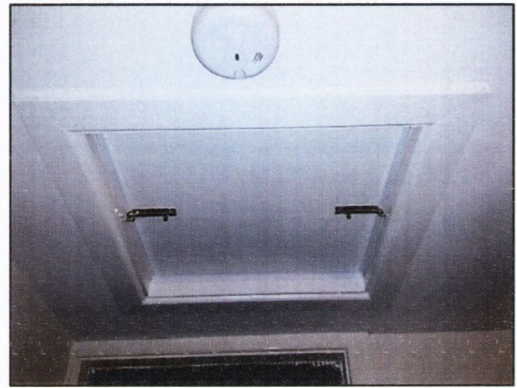
d) Attic hatch with holding down latches
