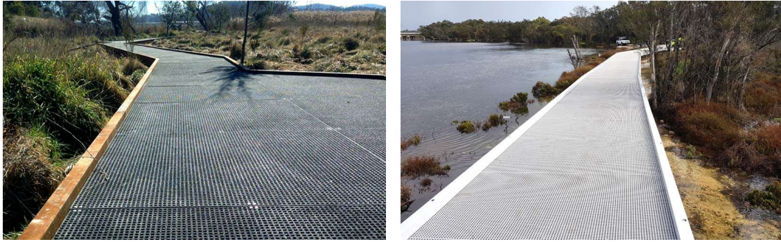
Fig 35: Imagery showing modular boardwalk systems (Archatrak)
