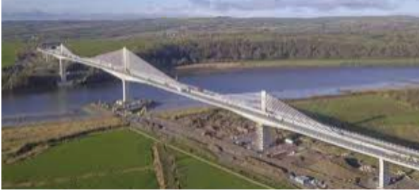
Figure 4: Cable Supported Bridges
