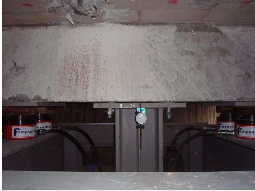
Fig 3.5.11.i. Jacks ready to take load with deflection gauge installed (Confidential Source, 2015).
