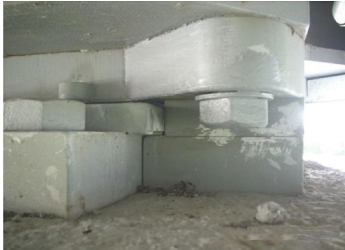
Fig 3.5.2.d. View of sliding bearing (Confidential Source, 2015).
