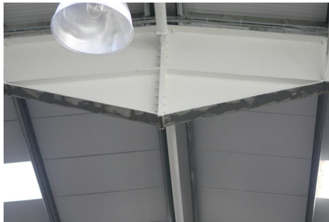
Fig 3.5.22.d. Portal ridge. (Confidential Source, 2015).
