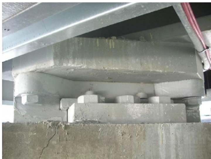
Fig 3.5.2.e. Alternative view of sliding bearing (Confidential Source, 2015).
