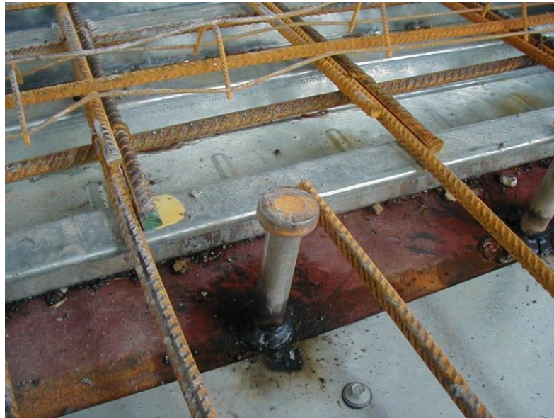
Fig 3.5.19.b. Photograph showing the stud welded to the steel beam using stick welding procedures. (Confidential Source, 2015).
