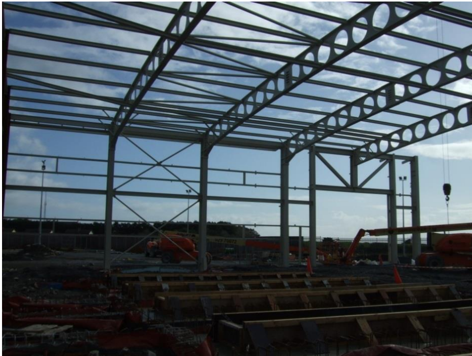
Fig 3.5.1.a. Photograph taken during steel erection showing the roller shutter door ope. (Confidential Source, 2015).
