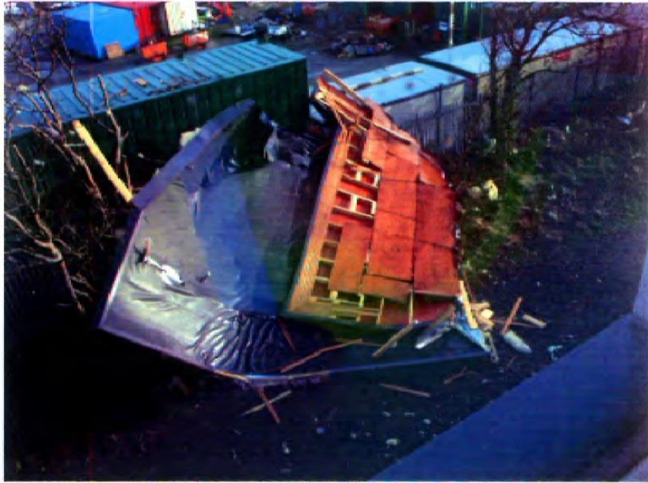
Fig 3.5.24.b. A section of roof landed in the car park. (Confidential Source, 2015). (note sections of lower plywood attached to upper joists.)
