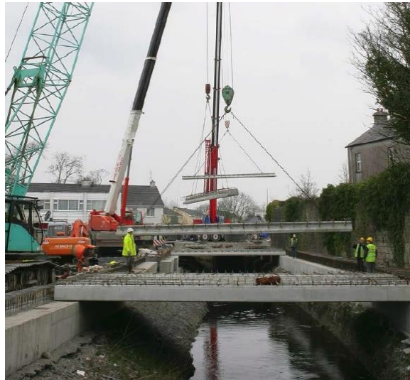
Fig 3.5.28.b. Lifting precast beams. (Confidential Source, 2015).
