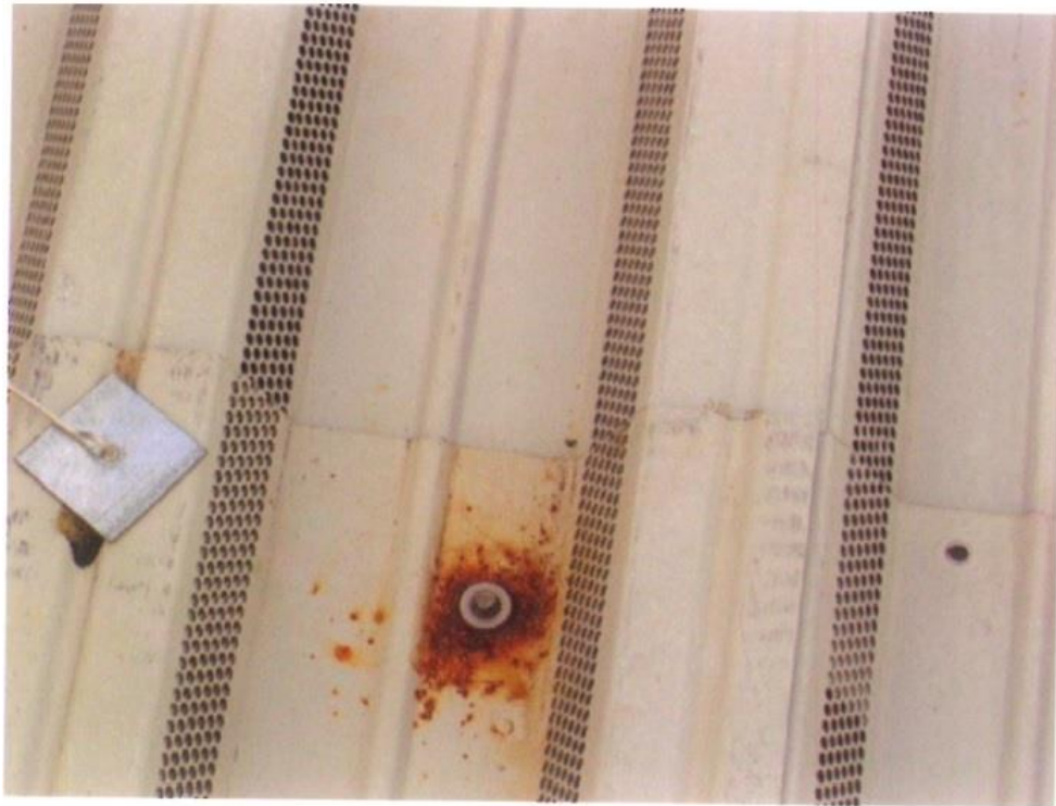
Fig 3.5.8.g. View of lower sheet. (Confidential Source, 2015).
