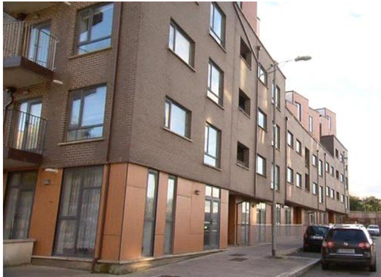
Fig 2.2.2.a Priory Hall (completed 2007) (Northern Sound, 2013)
