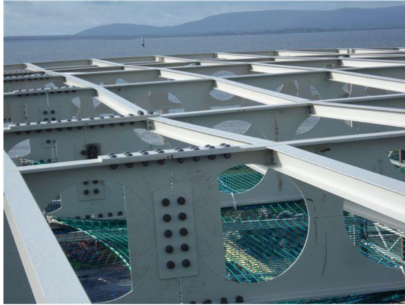
Fig 3.5.1.b. Photograph showing the sag in the castellated rafter. (Confidential Source, 2015).
