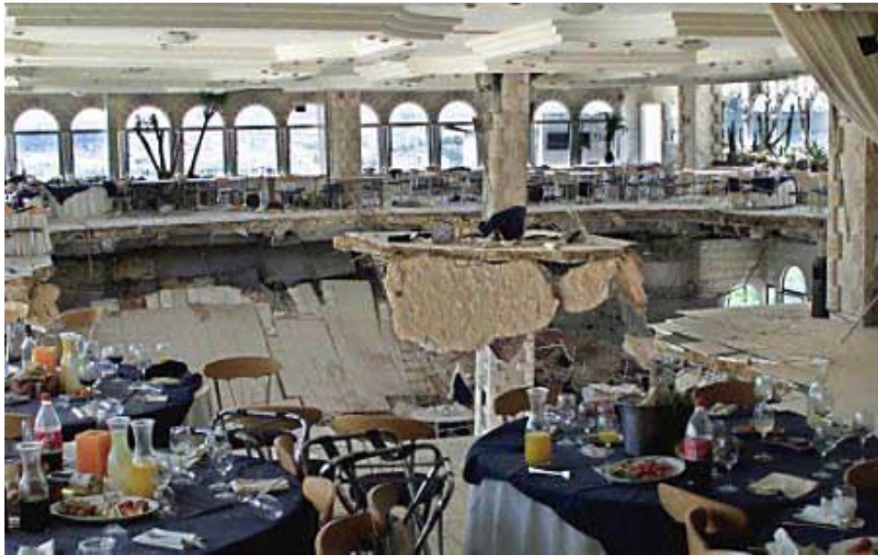
Fig 2.7.3.a Versailles Wedding Hall (Zailer Committee Report, 2002) (note the long spans and punching shear at column)
