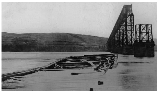
Fig 2.3.2.a Tay Bridge after collapse in 1879 (North British Railway Study Group 2016)
