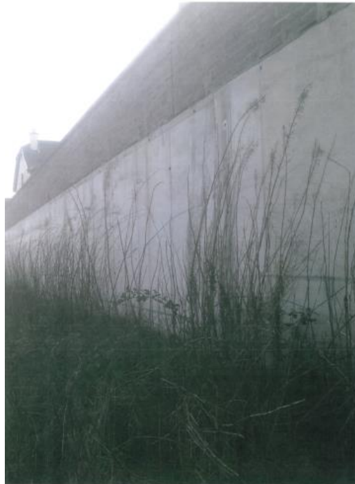
Fig 3.5.32.a. View of retaining wall (note house in the distance). (Confidential Source, 2015).
