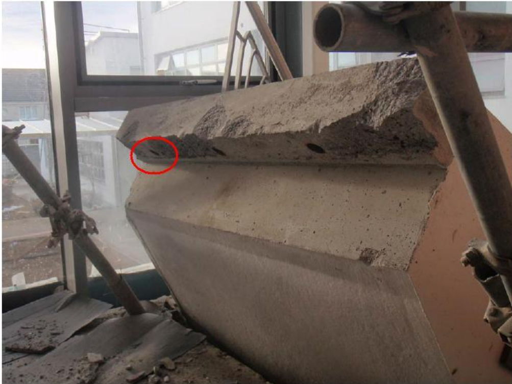
Fig 3.5.14.d. Detail at top halving joint (note: dowel hole). (Confidential Source, 2015).
