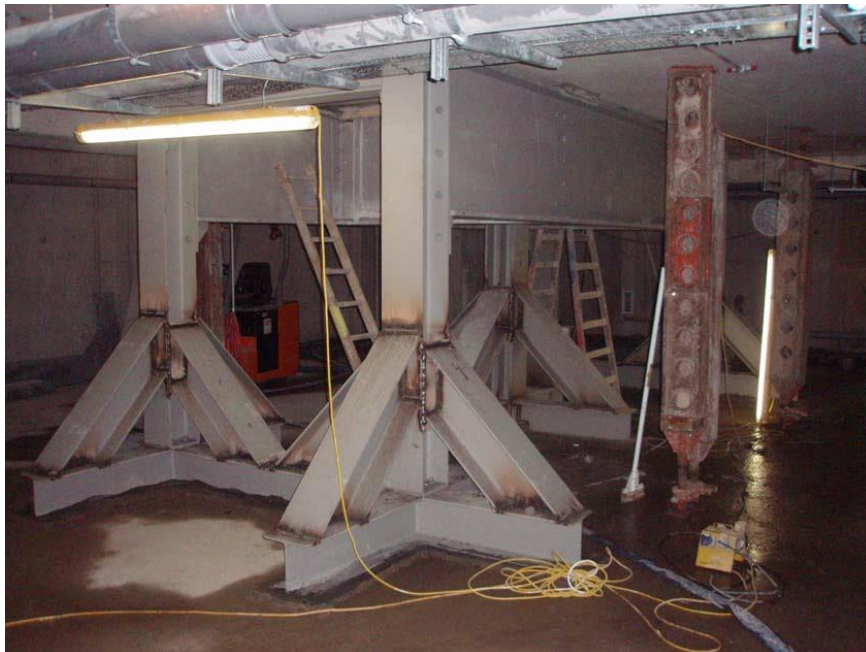
Fig 3.5.11.h. View at lower basement showing temporary propping (Confidential Source, 2015).
