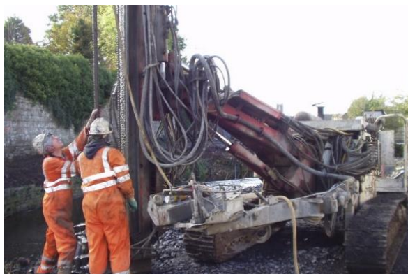
Fig 3.5.28.a. Mini-pile rig in use. (Confidential Source, 2015).
