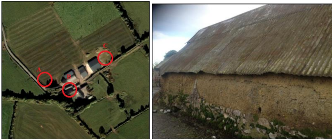
Figure 1: Right- Traditional earth building at Rhode, County Offaly. Left- Building location (B) with respect to earth pits both original (A) and current (C).
