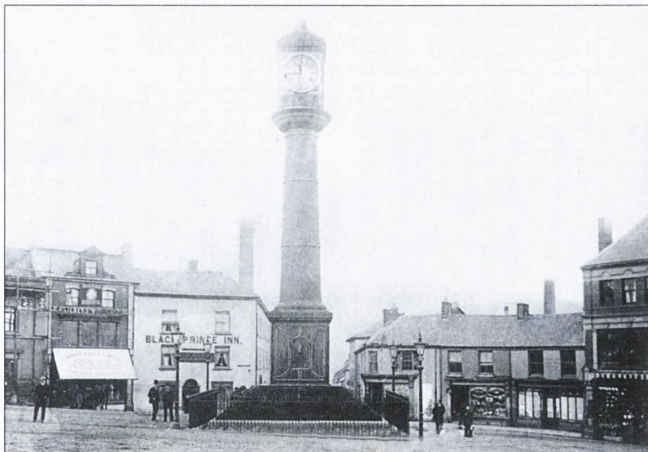
Figure 5.3.8: Photograph depicting the clock tower in 1908. From Philip Prosser, A Look at Old Tredegar in Photographs (Volume 2) (Abertillery: Old Bakehouse Publications, 1998), p. 28.
