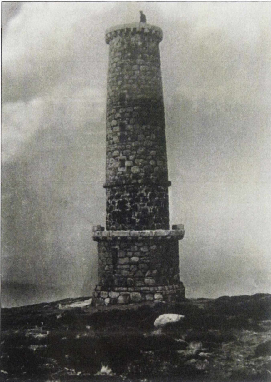
Figure 4.3.4: View of the Waterloo Monument showing climber at summit. From Ewart Library, Dumfries, GKd21(718), New Abbey: Waterloo Monument , (no date).
