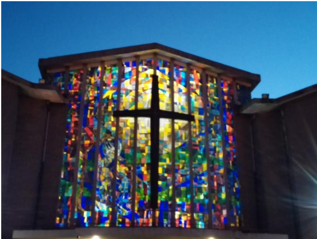
Figure 56. Exterior view of Church of the Annunciation, Finglas, Dublin.
