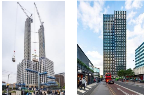
Figure 1. Partially completed case study building showing tied cores (left) and completed case study building (right)
