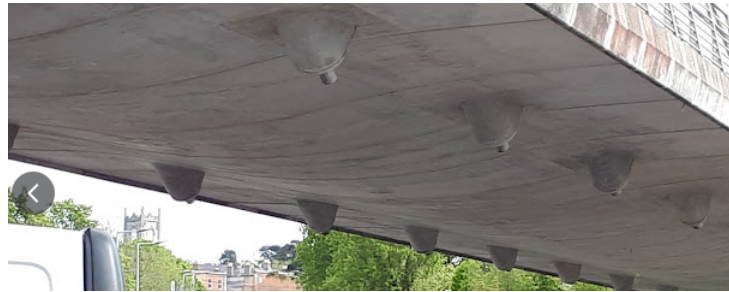
Figure 2.27. Cable anchorages protruding the deck of the William Dargan Bridge, Dublin, Ireland
