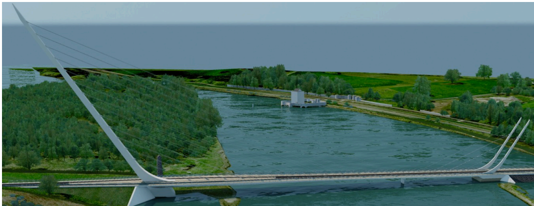
Figure 3.14. Future Narrow Water Bridge in Louth Co., Ireland 2
