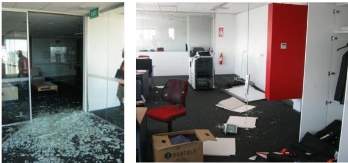
Figure 4-1 Non-structural damage after the 2011 Christchurch earthquake (Clifton and MacRae, 2013)
