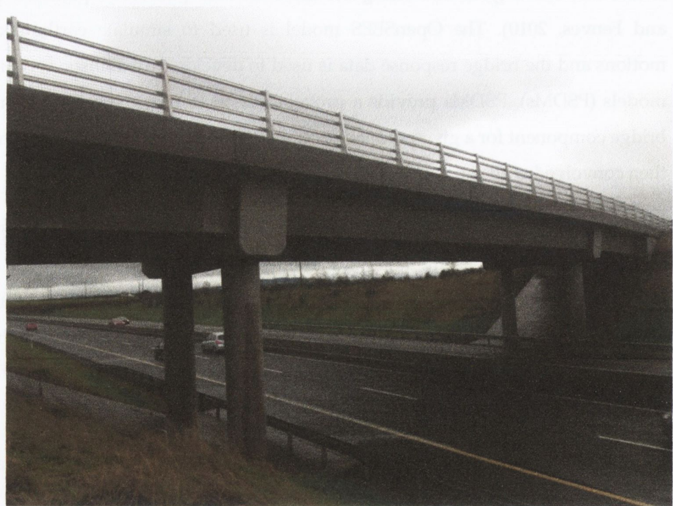
Figure 3.1 52m Three-span fully integral bridge
