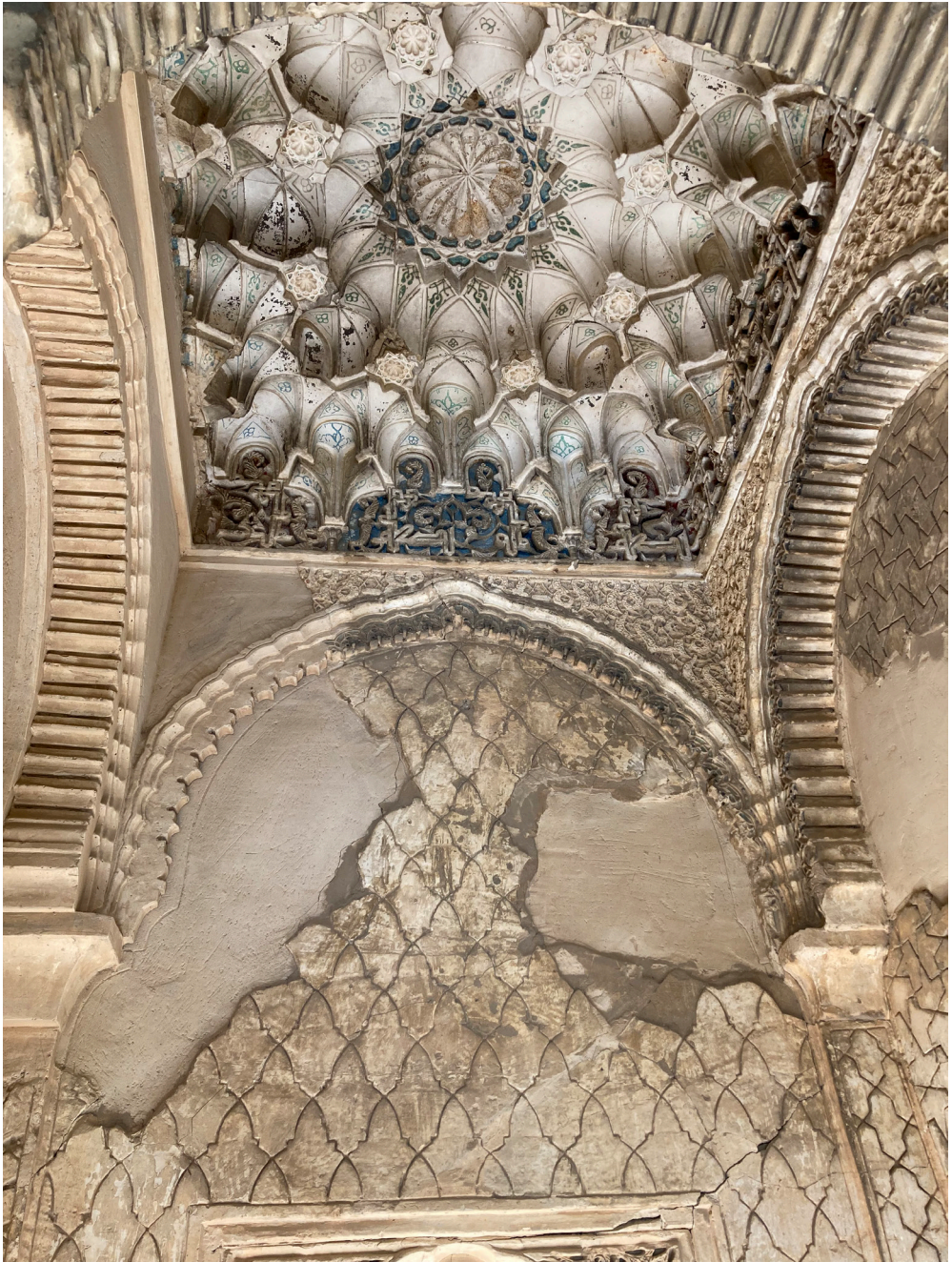
Figure 20.6 Detail of the Partial plaster ceiling. Photograph: Anna McSweeney.
