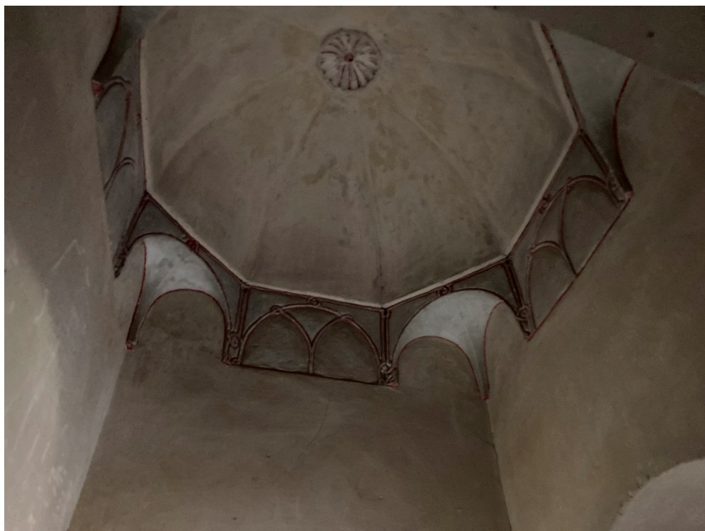
Figure 20.8 Detail of the Partal lower staircase plaster ceiling. Photograph: Anna McSweeney.
