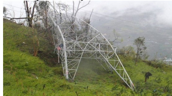
Figure 1. Typhoon Nepartak caused the power tower to collapse (Taipower, 2016)
