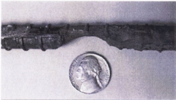
Figure 2.17 Reinforcing steel bar affected by pitting corrosion (Reis et al. , 2005)
