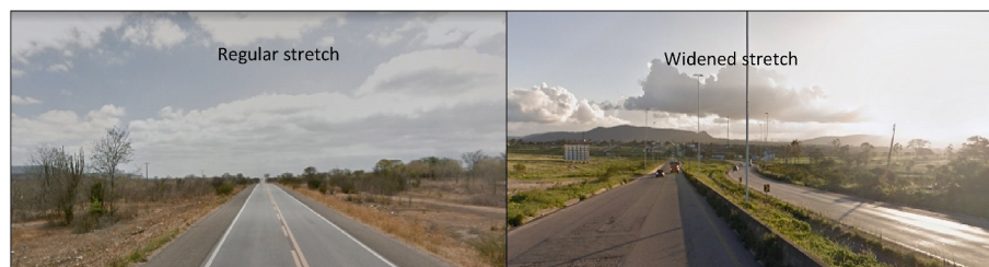
Fig. 1. Road BR-232 - The original motorway on the left with just two lanes, and the widened stretch with four lanes on the right (Source: Googlemaps Streetview).
