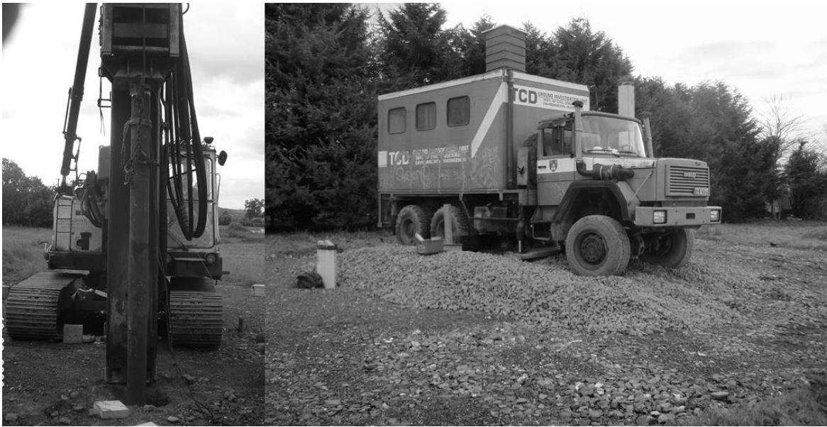
Fig. 5 (a) Pile driving and (b) Pile load testing at the Mortarstown site.
