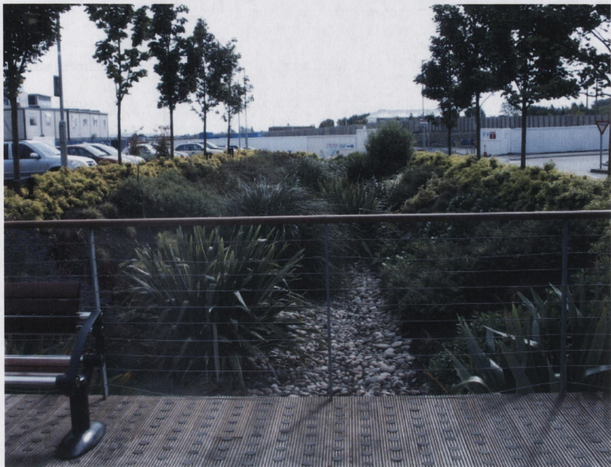
Figure 72: Swale in Pelletstown March 2010
