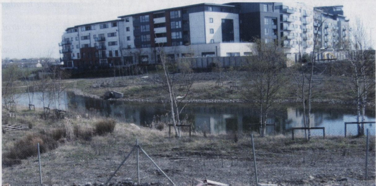
Figure 19: Retention pond Pelletstown North Dublin March 2010
