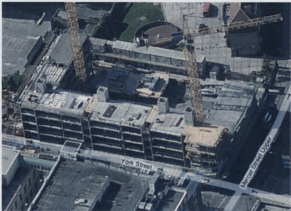
Figure 56: Aerial Photo of Construction (bing maps 2009)
