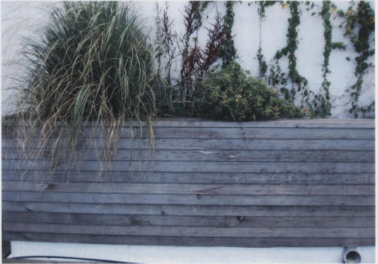
Figure 59: Roof Garden (part of Green Roof) July 2010
