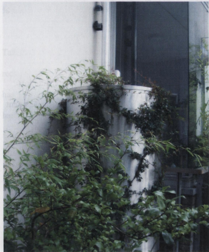
Figure 58: Rain water Harvesting Tank York Street July 2010
