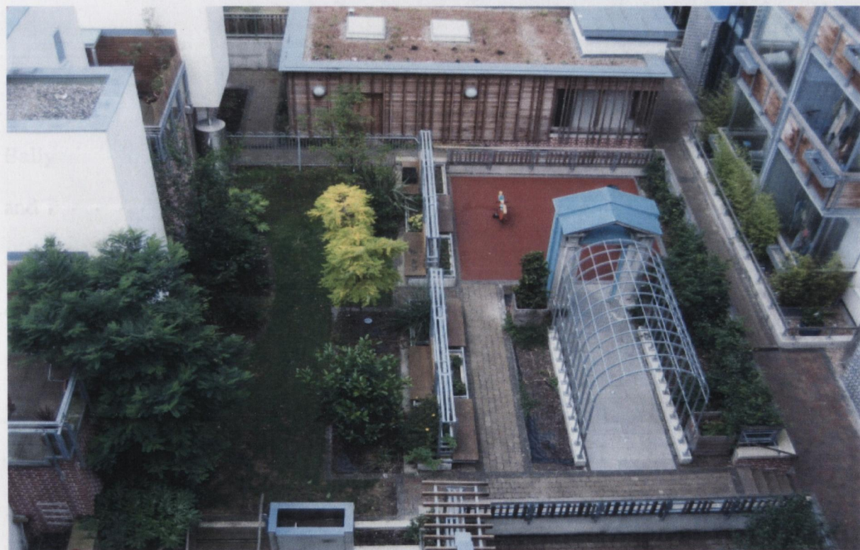
Figure 61 Courtyard above car park York Street July 2010
