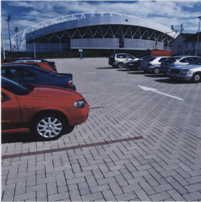
Figure 12 permeable paving Thomond park Limerick ( tobermore 2010)
