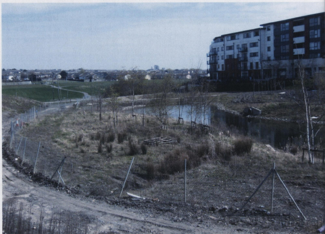
Figure 70: Retention pond in Pelletstown March 2010
