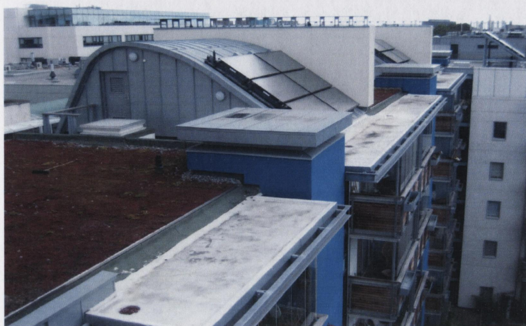
Figure 51: Roof York Street July 2010
