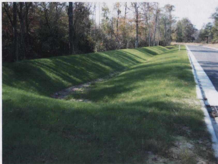
Figure 10: Swale North Carolina USA (Thomas engineering 2010)
