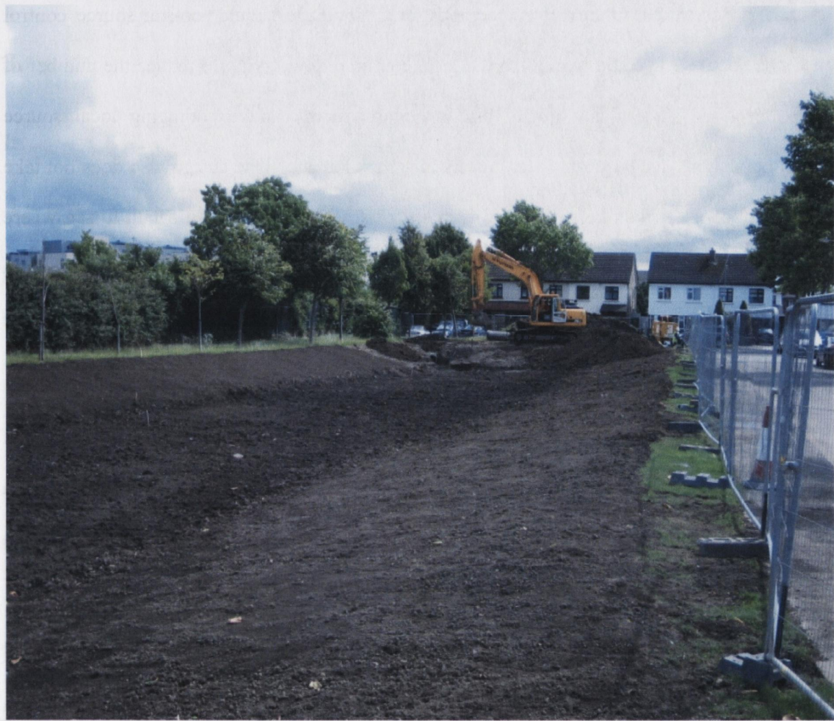
Figure 31 Construction of Swale 1 at Glendhu Park
