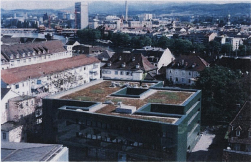
Figure 16 Extensive green roof in Basel Switzerland (DCC Green roof policy 2008)
