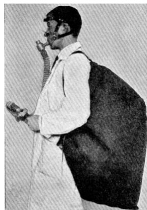
Plate 1.1: A portable Douglas bag system for exercise testing (Hill et al. , 1924).
