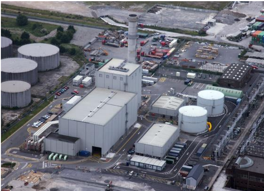
Figure 1-2: 410MW Combined Cycle Gas Turbine, Dublin Bay Power
