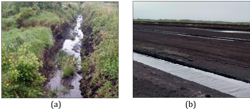
Figure 1.9: Artificial drainage on peat extraction sites showing (a) drain on a cutover site with growth and infill and (b) drain on industrial bare peat site (Co. Roscommon).
