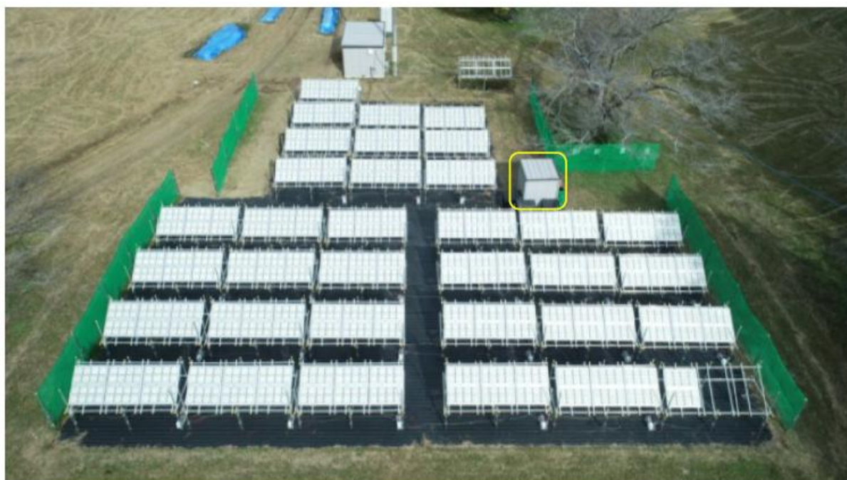
Figure 1.9: An aerial photograph of the 100 m 2 scale photocatalytic solar hydrogen production system consisting of 1,600 reactor panel units and a gas separation unit (indicated by the yellow box). Reproduced with permission from Nishiyama et al. 55
