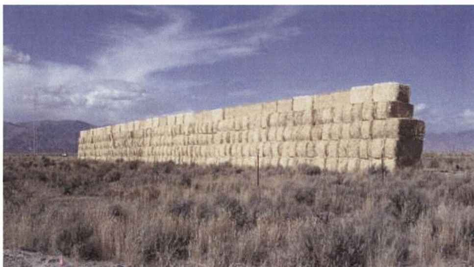
FIGURE 2.9. STRAW STACK CONSTRUCTED AS A ROADSIDE NOISE BARRIER (FINN ET AL., 2010).
