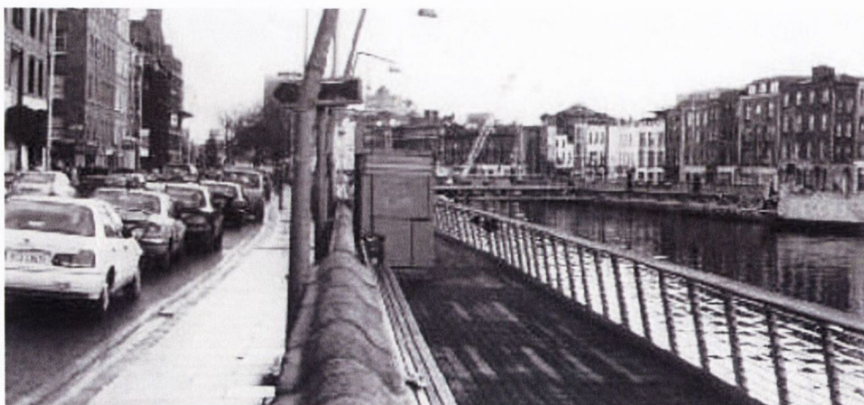
FIGURE 2.3. RIVER LIFFEY BOARDWALK IN DUBLIN, IRELAND (KING ET AL., 2009).
