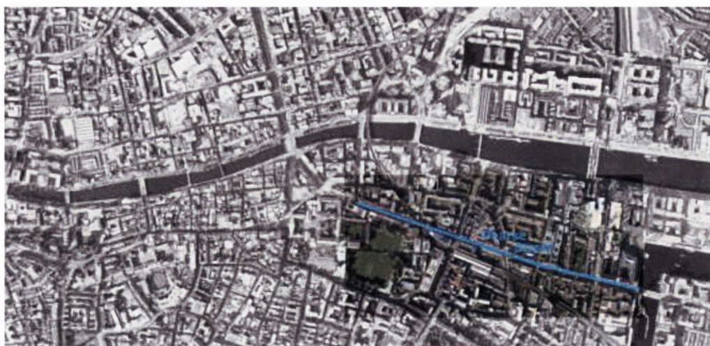
FIGURE 6.1. PEARSE STREET IN DUBLIN CITY CENTRE (GOOGLE EARTH, 2012).
