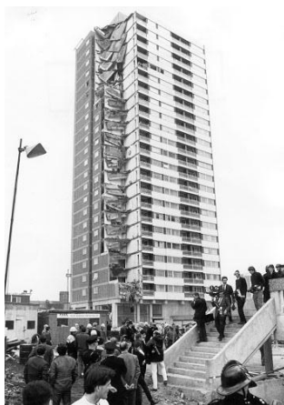
Figure 1. Ronan Point collapse.
