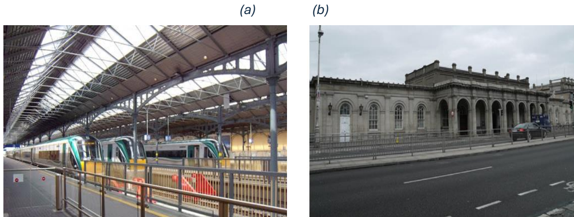
Figure 3.2. (a) Terminal platforms at Heuston. (b) Heuston south entrance at St. Johns Road.
