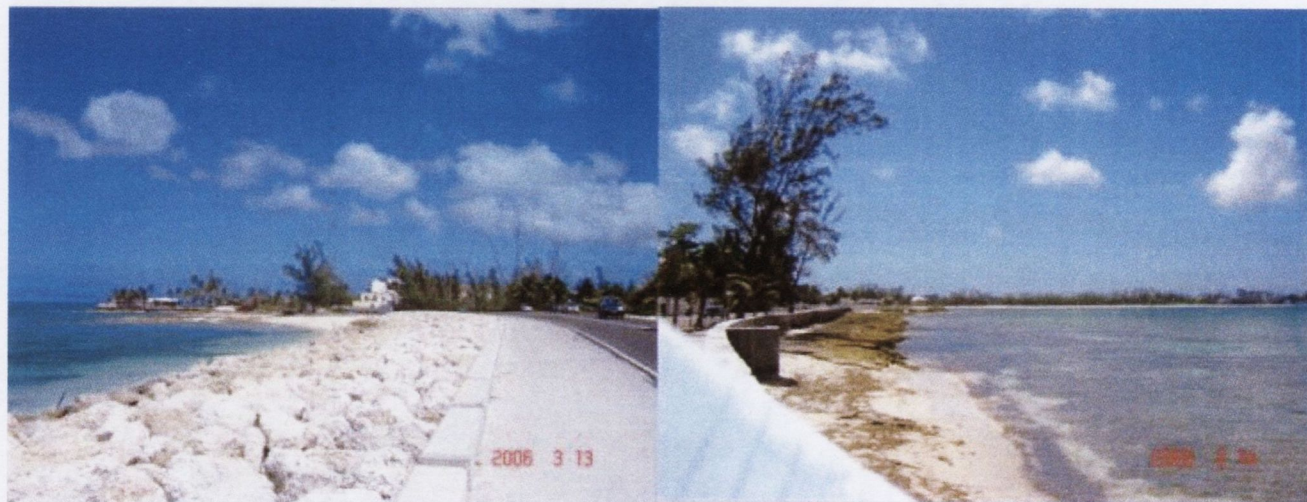
Figure 3.7. Sea wall construction in New Providence Island leading to beach erosion.
