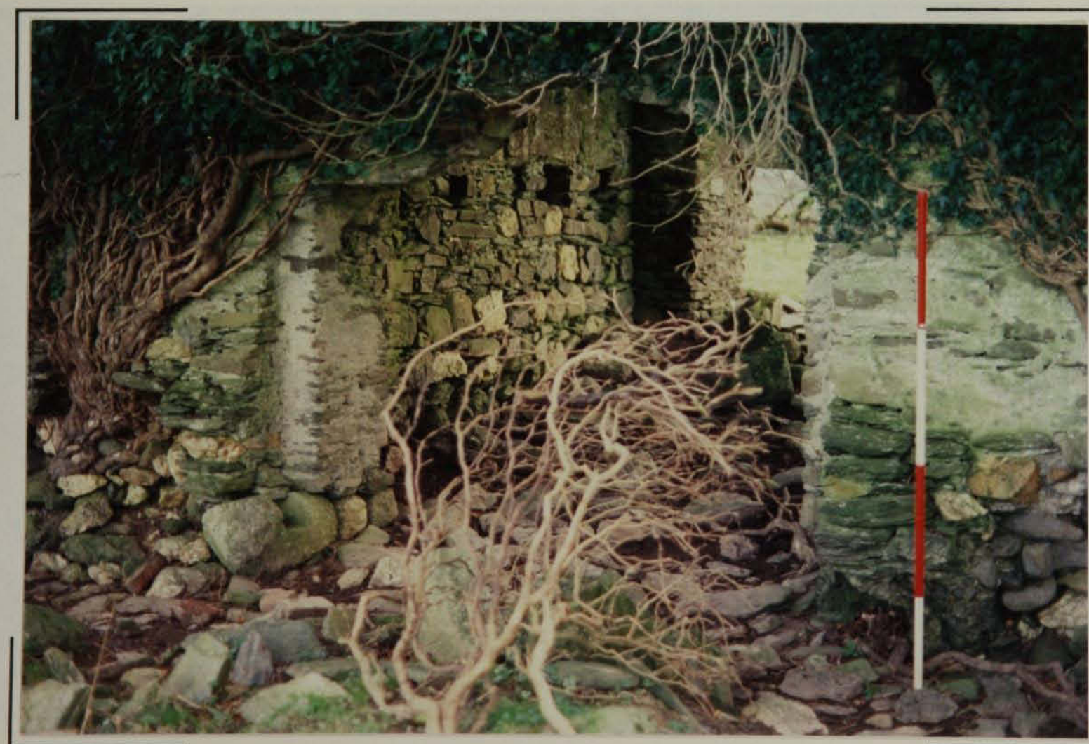
Plate 4.23a Rebate in Wall Talus and base stone, both indicate a drawbridge at Borris (#5).
