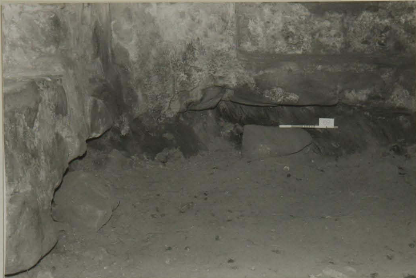
Plate 4.17 Foundation of boulders on natural rock outcrop. (Tracystown - #69)
