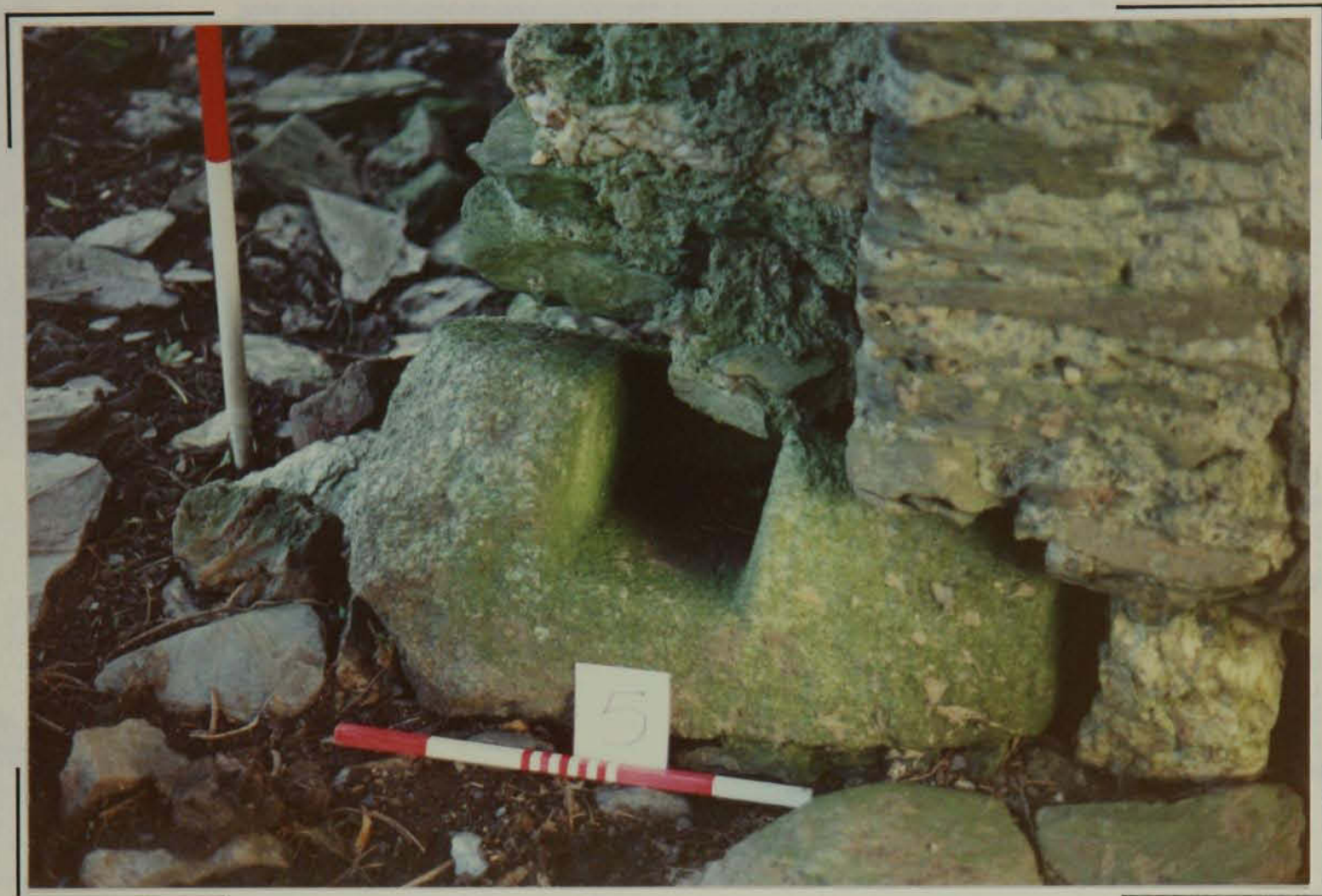
Plate 4.23 Stone suitable for horizontal hinging mechanism of drawbridge, Borris Castle.
