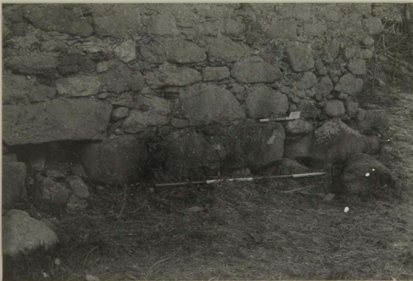
Plate 4.17a Boulders used as "foundation" at Tracystown (exterior view).
