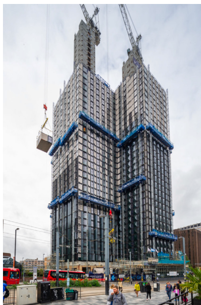
(a) During construction
