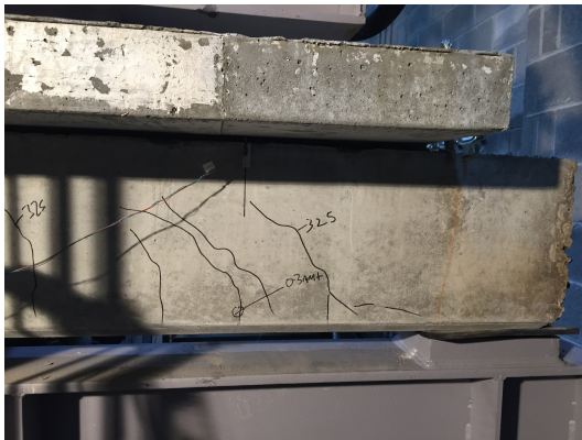
(c) PTB1-3 Cracking at 325 kN
