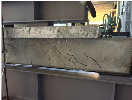
(c) PTB1-2 Cracking at 300kN
