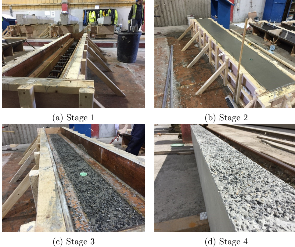
Figure 3.3: TB1-2, TB1-3 and TB1-4 Manufacturing Stages
