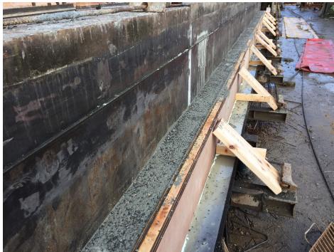
(c) Finished Beam
