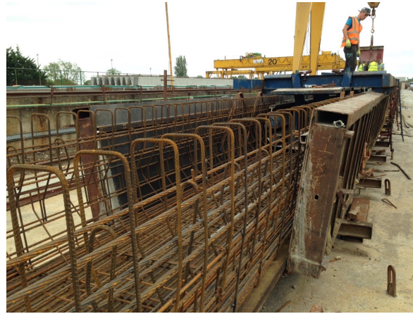
Figure 2.13: W Beam being poured in a precast factory
