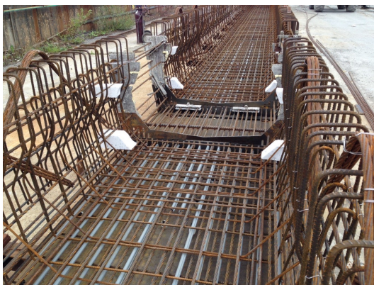
(a) Interface Shear Links At Beam Ends Prior to Concreting
