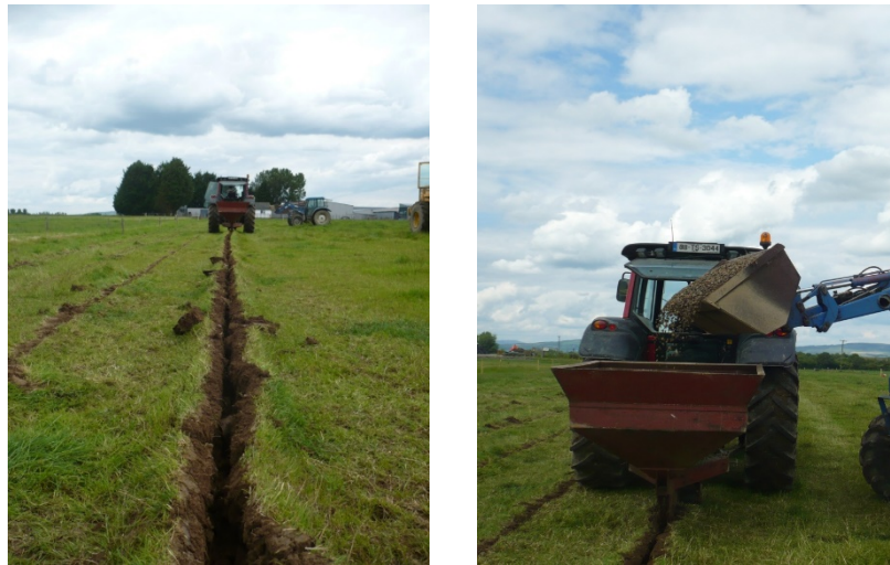
Figure X.6. Gravel mole drainage
