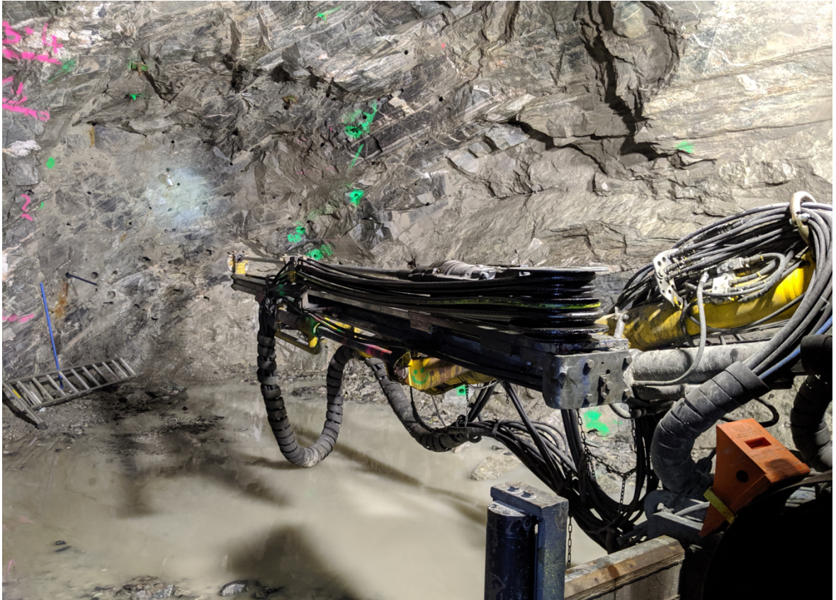
Figure 8.7. Underground drilling at Cononish (Scotgold Resources Limited, 2020b)
