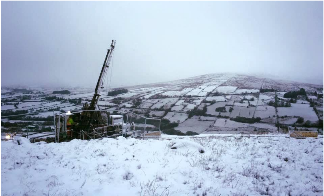
Figure 3.9. Drilling in the Sperrin Mountains at Curraghinalt, January 2016 (photograph by author).
