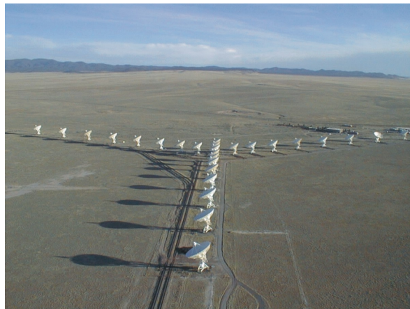
Figure 1.13: The VLA in its closest configuration, the D configuration. Credit: NRAO/AUI/NSF. Licensed under CC BY 3.0 ( https://creativecommons.org/licenses/by/3.0/ ).
