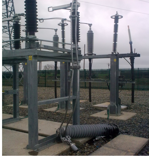
Figure 2: Example of a picture taken by one of the worker and sent as part of a near miss report on the failure of 110 kV cable sealing end
