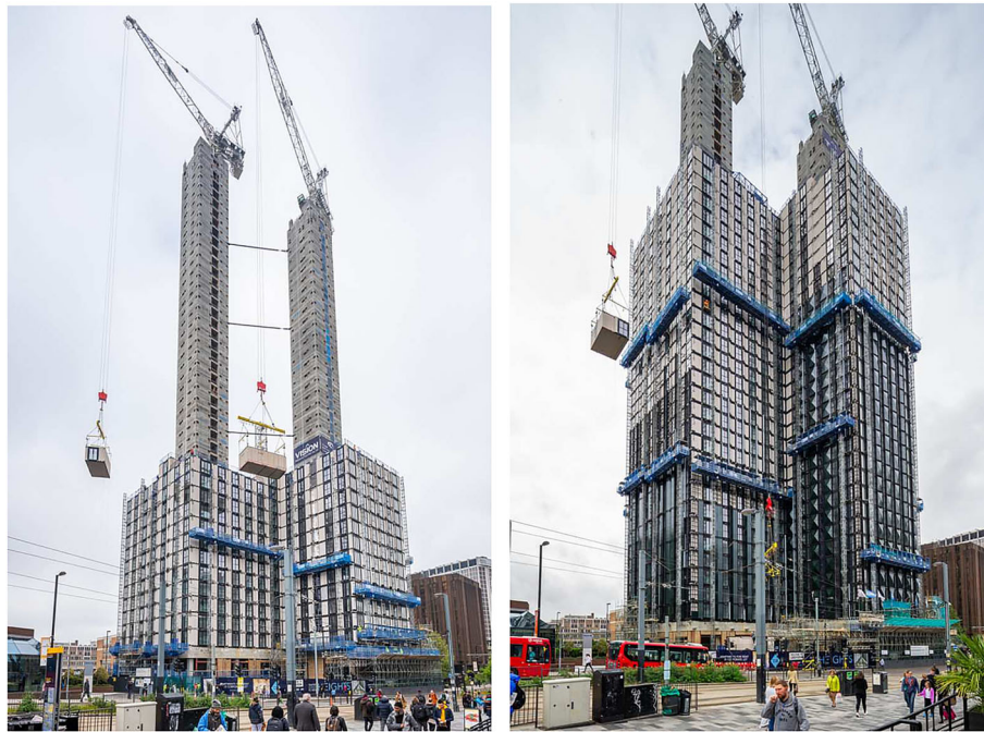
FIGURE 4 The Ten Degrees building in Croydon, London, pictured at two points in time during module installation. It can be seen how the structure consists of volumetric modules stacked around two RC cores. 32
