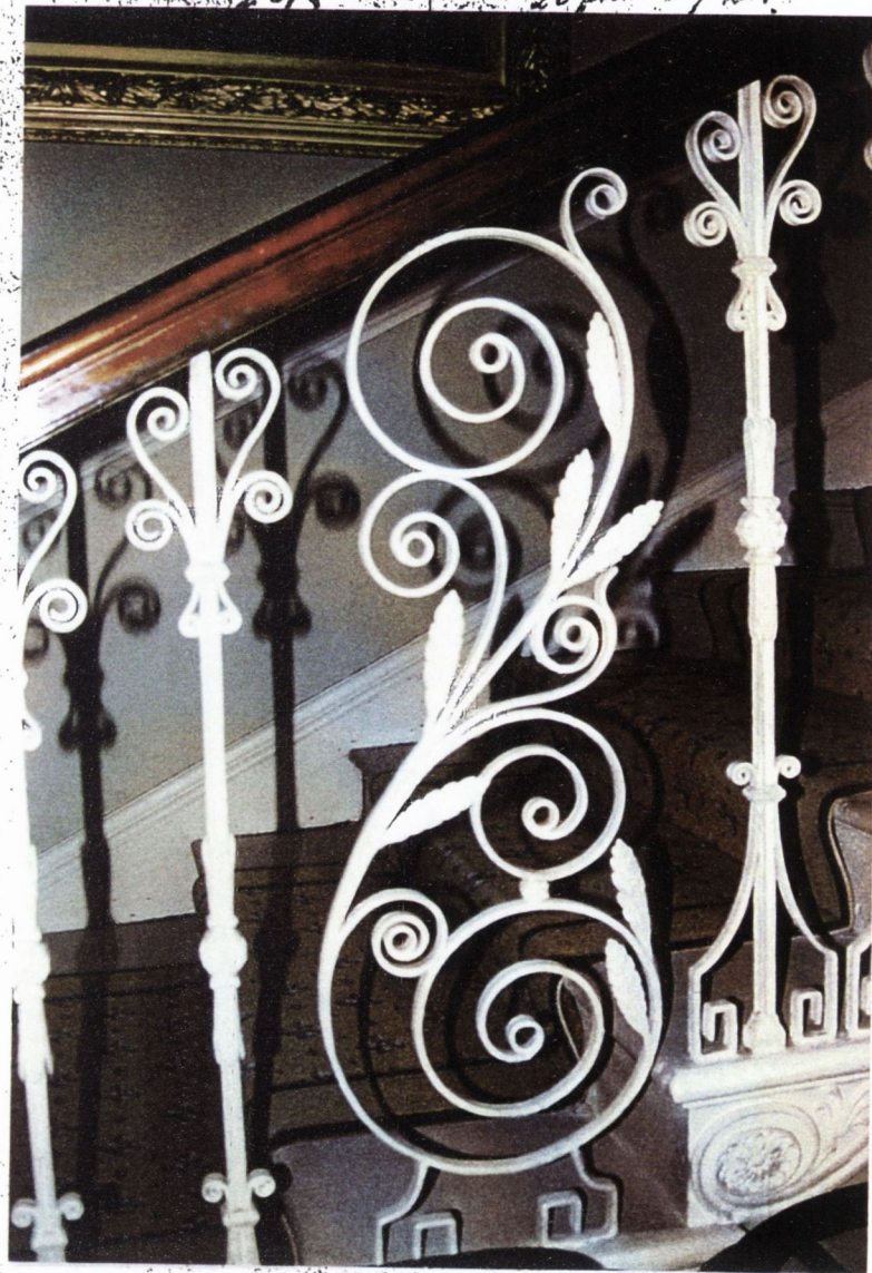
Plate 57. Recent photograph of Caledon Staircase balustrade
