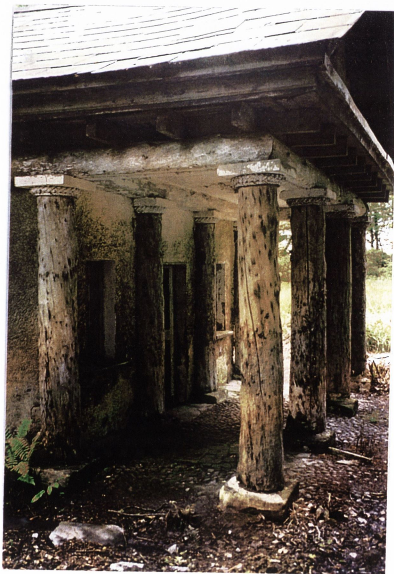
Plate 46. Belline Lodge, showing timber architrave, timber modillions and stepped cornice
