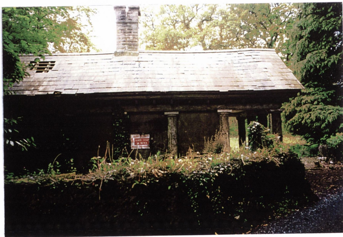
Plate 48. Side view of Belline lodge, showing semi-engaged rustic columns
