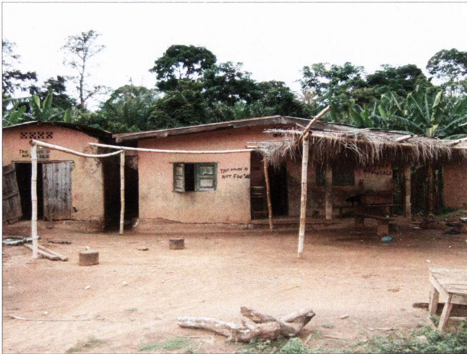
Plate 2.2 Typical village house with concrete walls and corrugated iron roof (Photo by: Patrick Kirwan)
