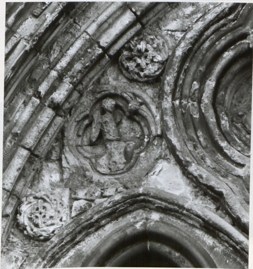
Plate 109: St Canices cathedral, Kilkenny. Detail of West doorway showing censing angels.
