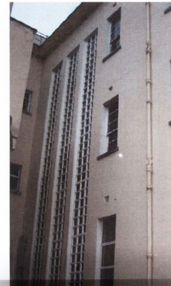
Figure 2.7, exterior stairwell glazing
