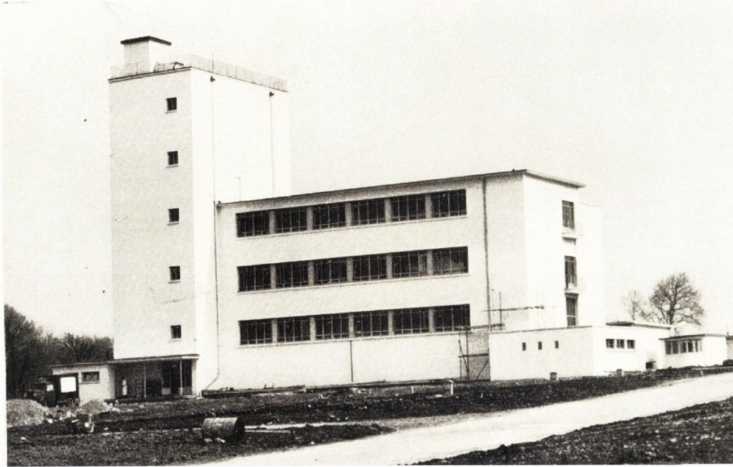
Figure 2.79 (upper left), boiler house
