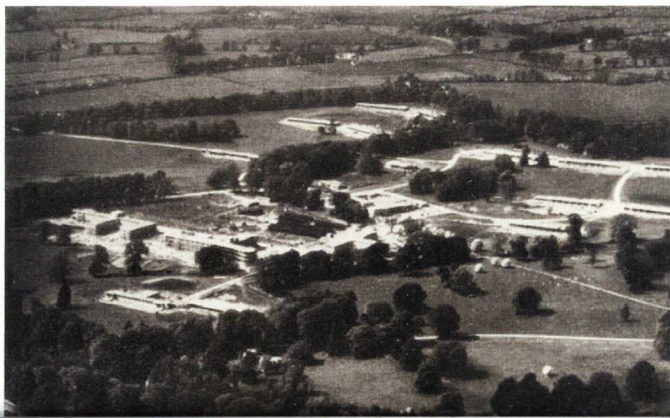
Figure 2.74 (left), aerial view
