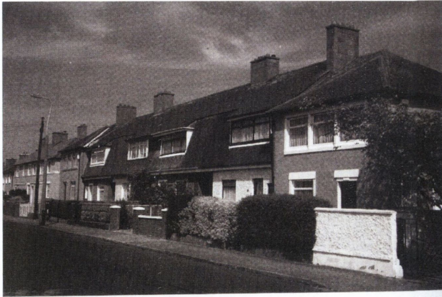
Figure 3.74 right , postcard view of Ferguson Road, housing on Drumcondra Estate, 1925-27, Horace O'Rourke (possibly Herbert Simms involved)
