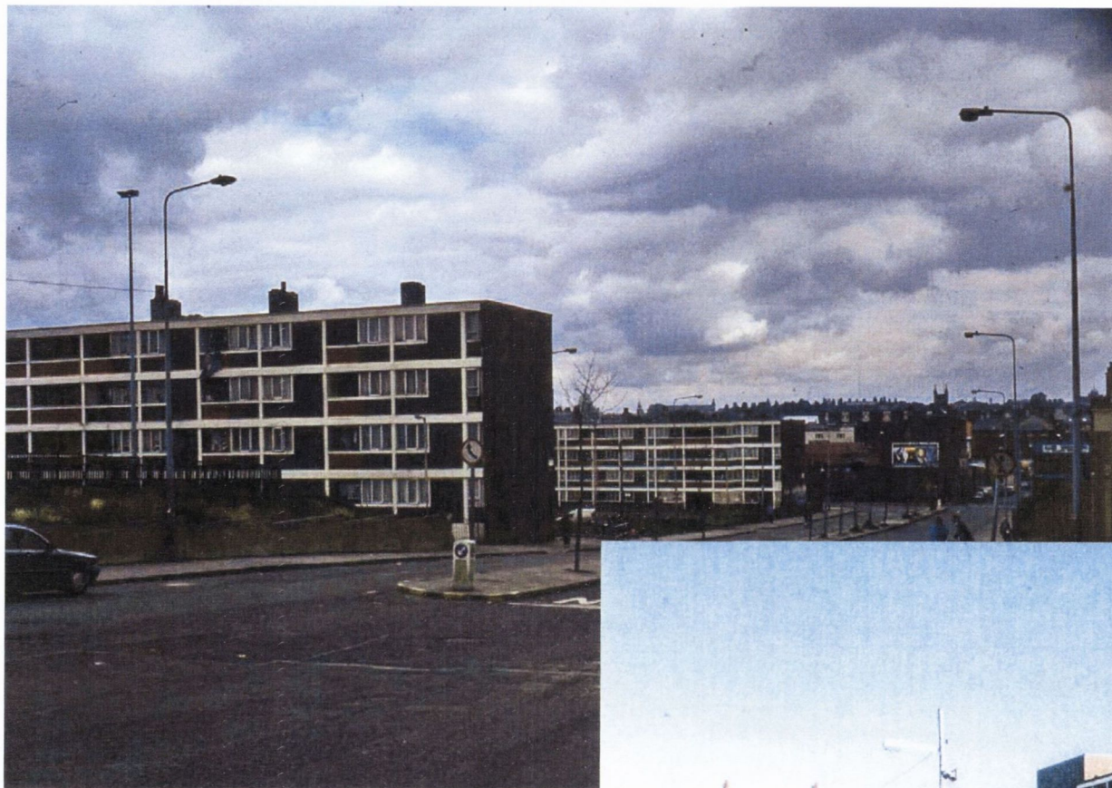
Bridgefoot Street scheme before demolition, c.2003:
