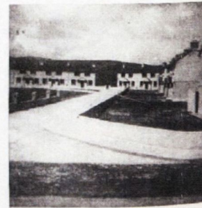
Cahir Housing Scheme— Tipperary (S.R.) County Council.
