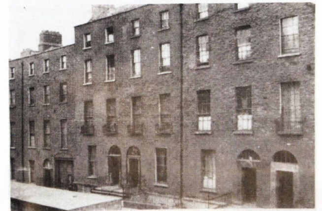
FRONT ELEVATION, PRIOR TO RECONDITIONING, OF HOUSES IN GARDINER STREET
