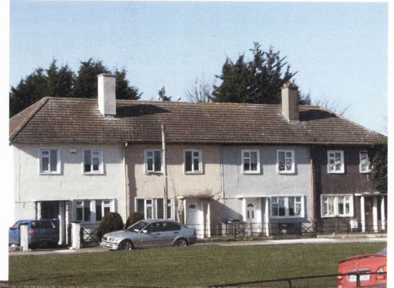
Figures 3.142 – 3.145 : the ORLIT prefabricated house at Crumlin, Captain's Avenue extension, 1948-1950, extant 2010 (photos: author's own)
