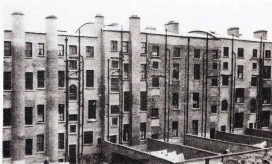
RERE ELEVATION, AFTER RECON- DITIONING, OF FOUR-STOREY HOUSES IN GARDINER STREET.
