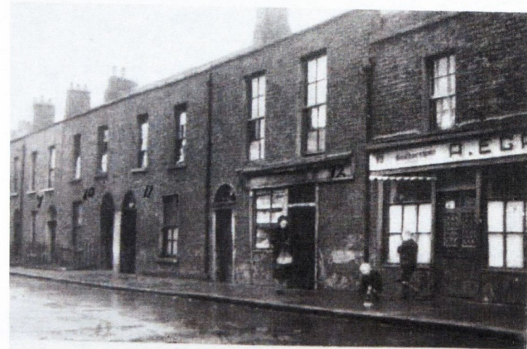
FRONT ELEVATION, PRIOR TO RECONDITIONING, OF TWO-STOREY HOUSES IN GLOUCESTER PLACE.
