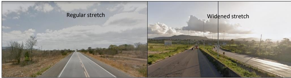
Figure 4.1: Road BR-232 - The original motorway on the left with just two lanes, and the widened stretch with four lanes on the right (Source: Googlemaps Streetview)
