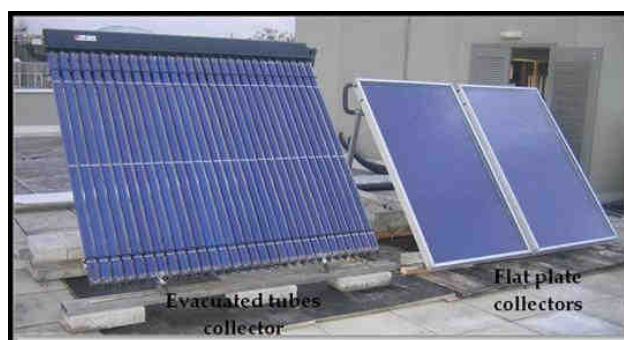
Fig. 1. Evacuated tube and flat plate collectors
